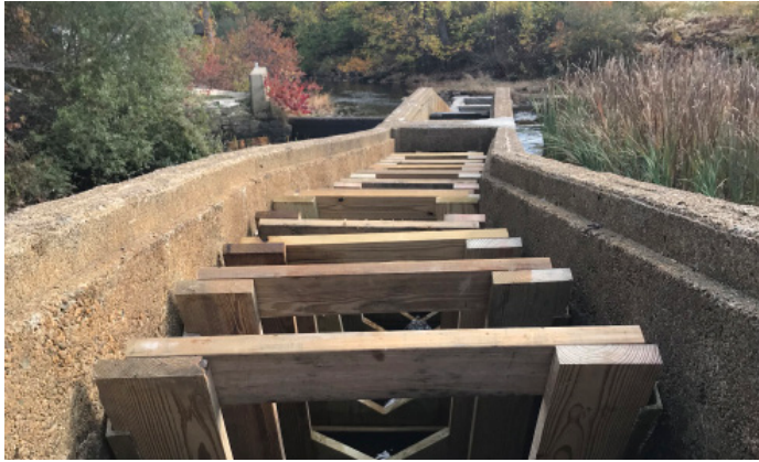
New Baffles at Indian Head River, Pembroke. October 2020.
