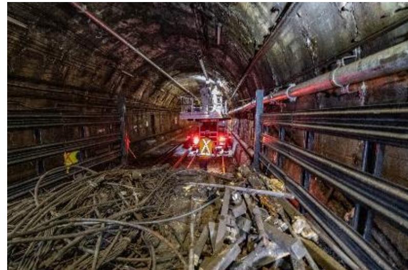
Blue Line Cable Removal
