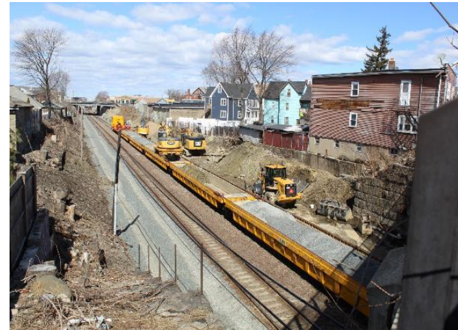
Project's Multi-Purpose Machine delivering railbed material to the narrow corridor (Jan. 2020)
