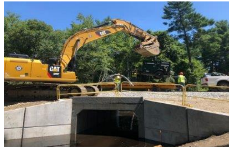
New Culvert in Freetown, MA
