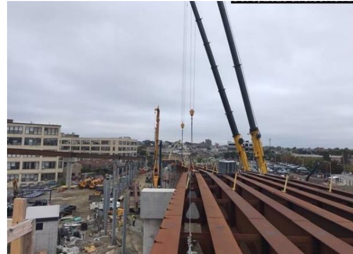
Final steel structure for GLX viaduct being installed (Oct. 2020)
