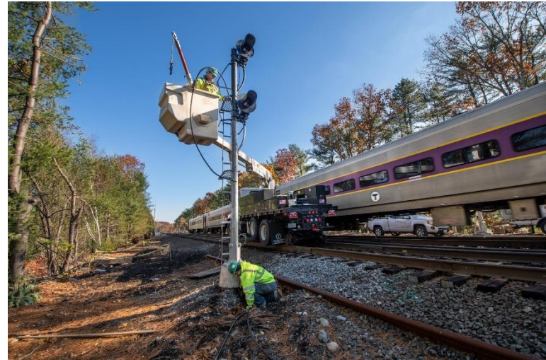
LED signal light installation as part of PTC upgrades
