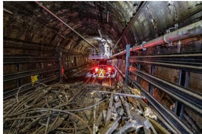
Blue Line Cable Removal
