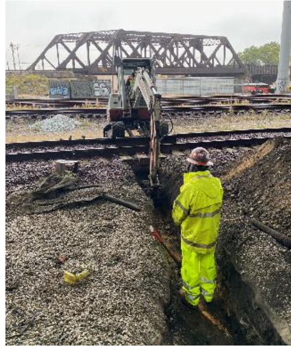
North Station Track and signal installation of 2-way conduits
