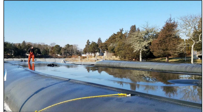
Bourne Pocasset River Dredging Project - Geotextile Bags Used for Dredged Material Disposal
