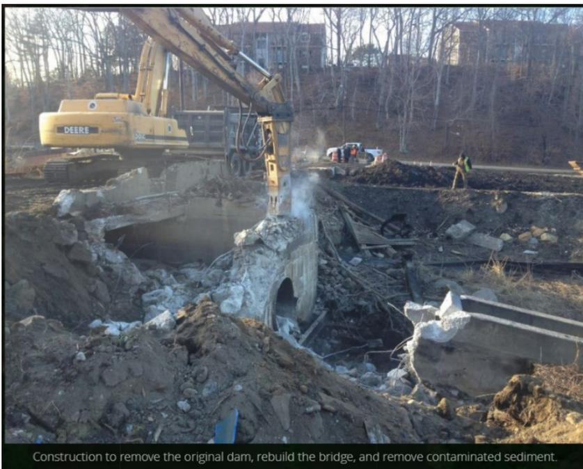
Construction to remove the original dam, rebuild the bridge, and remove contaminated sediment.
