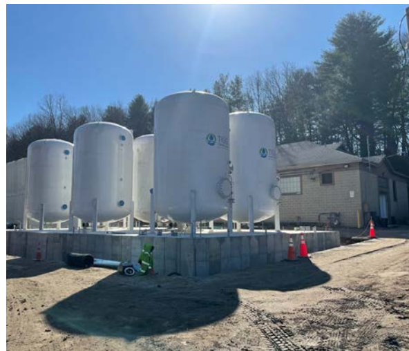
Vessels at Chestnut Street PFAS Treatment System
