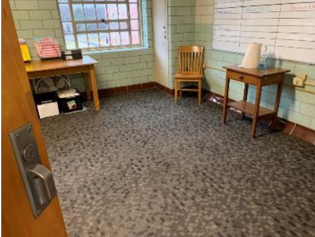
ACM 9" x 9" gray with green streak floor tile beneath carpet
