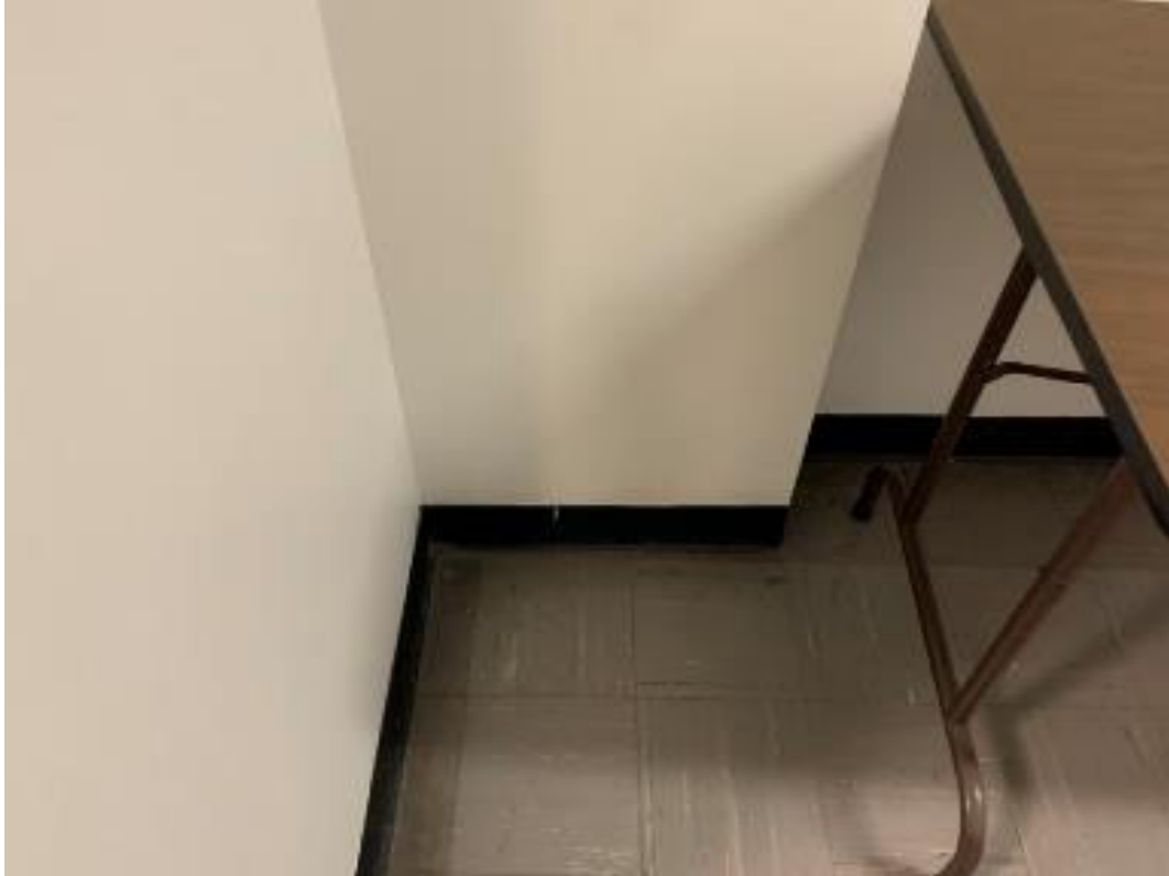
Wall base molding and associated adhesive
