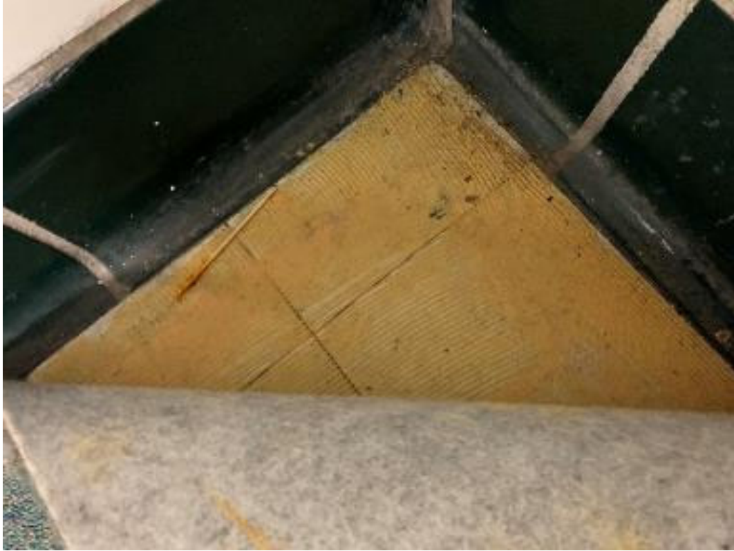
ACM 9" x 9" floor tile beneath carpet in hallway
