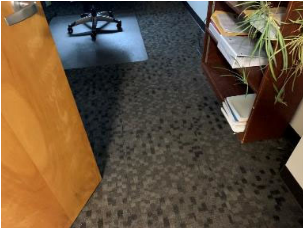
Carpet with ACM 9" x 9" gray floor tile beneath
