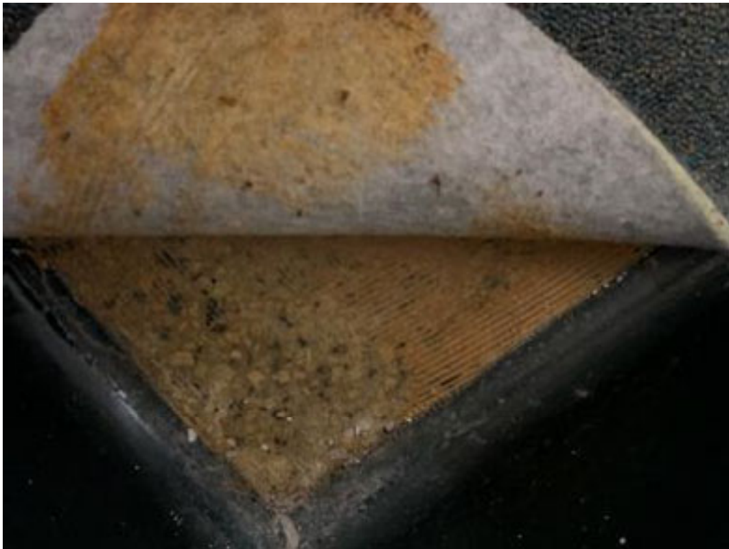
Terrazzo flooring beneath carpet in hallway
