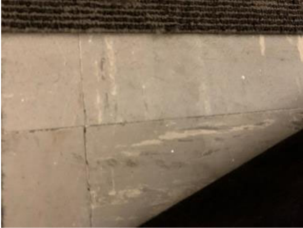
ACM 9" x 9" gray floor tile beneath carpet
