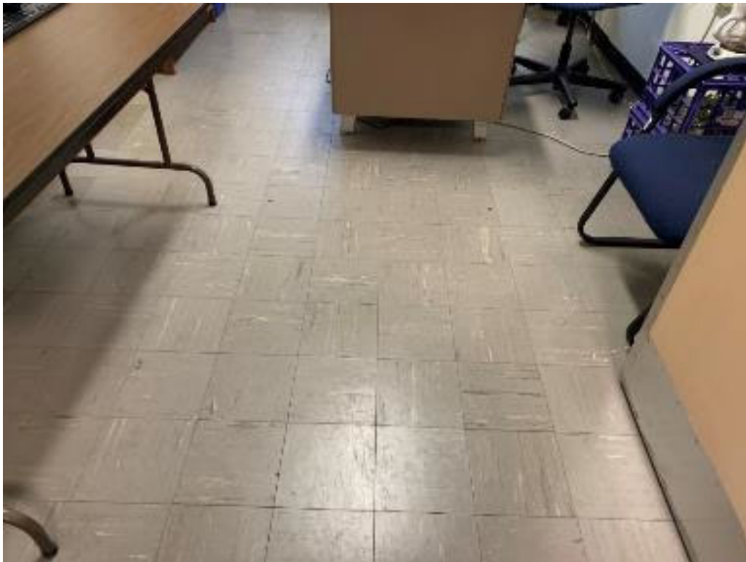
ACM 9" x 9" gray floor tile and associated black mastic
