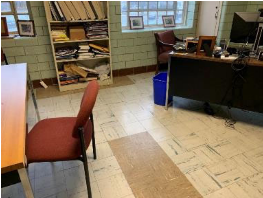
Typical glazed block wall
