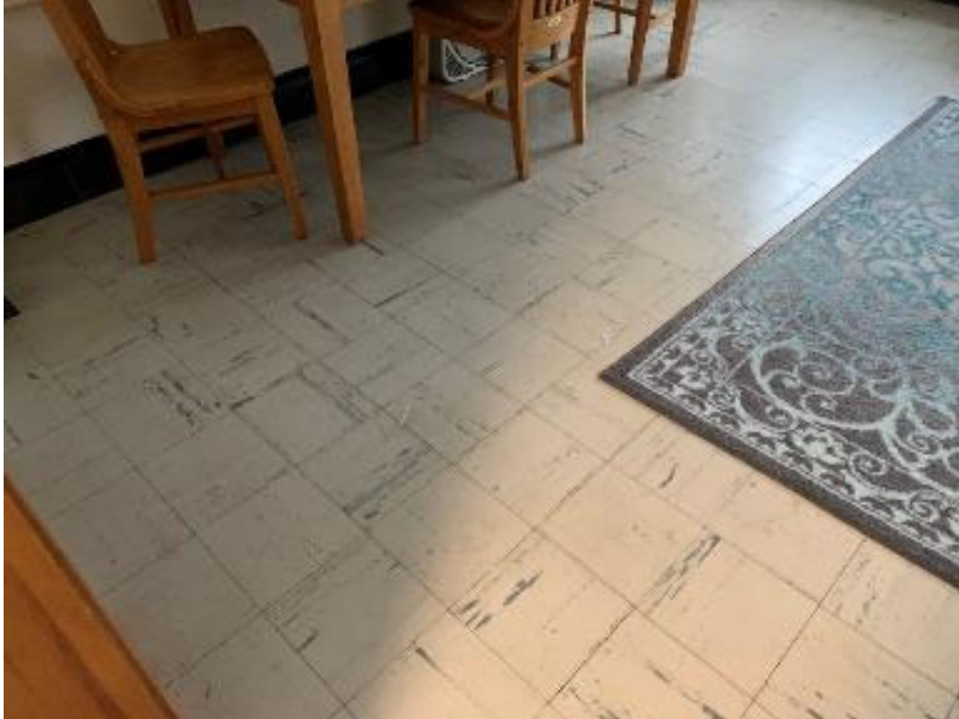
ACM 9" x 9" gray with green streak floor tile
