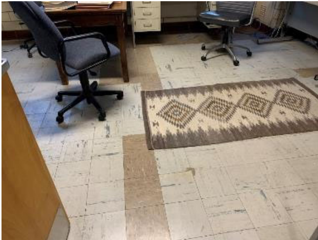
ACM 9"x 9' Gray with green streak floor tile and ACM brown replacement tile
