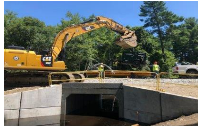
New Culvert in Freetown, MA
