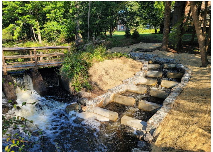
Figure 48. The new fishway at Howlett Brook in Topsfield.
