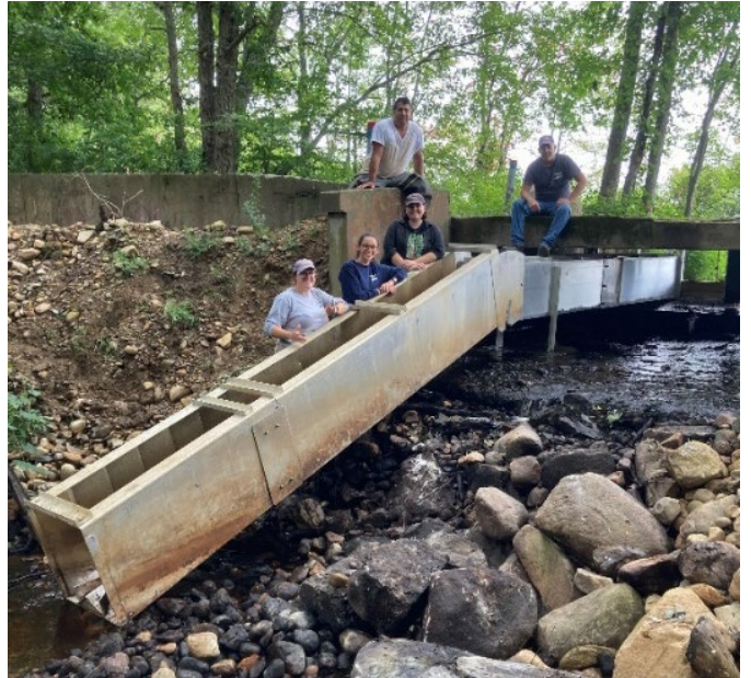
Figure 47. The new fishway is fabricated at the Fishway Crew shop in New Bedford (left) and installed (right) at the Stump Brook Bog Reservoir Dam, East Bridgewater.
