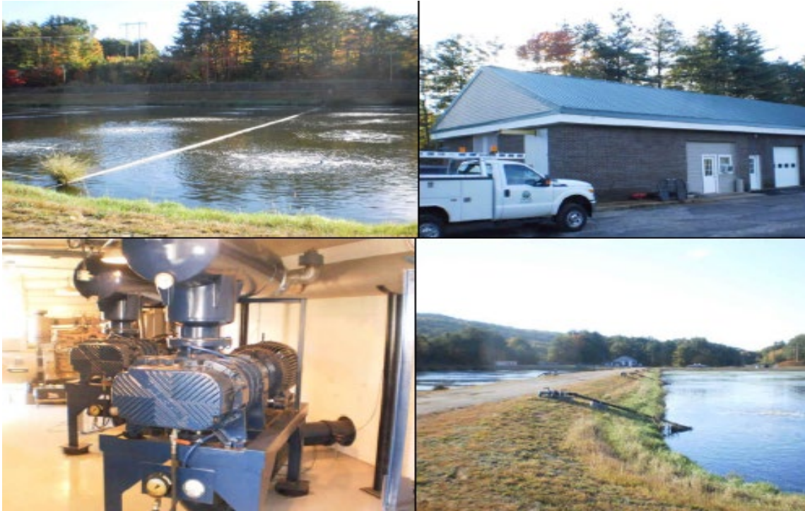
SELECTED IMAGES OF THE ASHLAND WASTEWATER TREATMENT FACILITY
