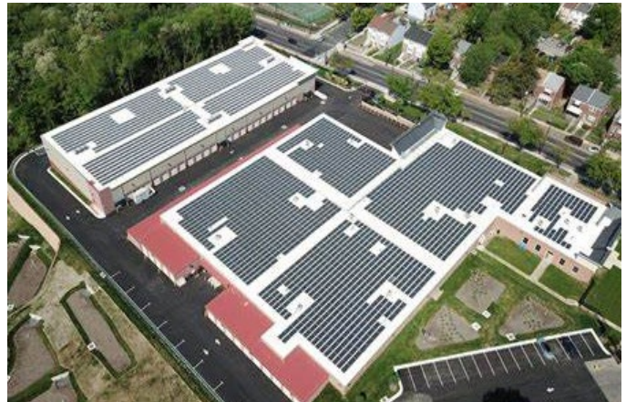
MSEC GRANT RECIPIENT, THE CITY OF CAMBRIDGE, INSTALLED A 42.64 kW SOLAR ARRAY WHICH RESULTS IN A REDUCTION OF GREENHOUSE GAS EMISSIONS AND LOWER ELECTRICITY BILLS.
