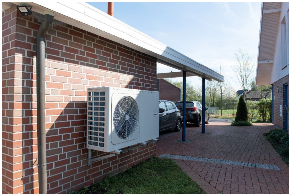
AIR SOURCE HEAT PUMP INSTALLATION AT A NEW HOME DEVELOPMENT
