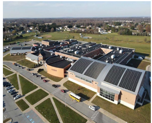
SOLAR INSTALLATION - BIRD VIEW OF ST. GEORGES VO-TECH
