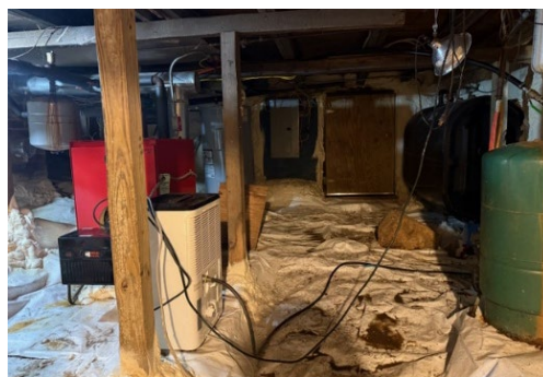
EQUIPMENT USED FOR RESTORING AND WEATHERIZING MR. SERKIN'S BASEMENT
