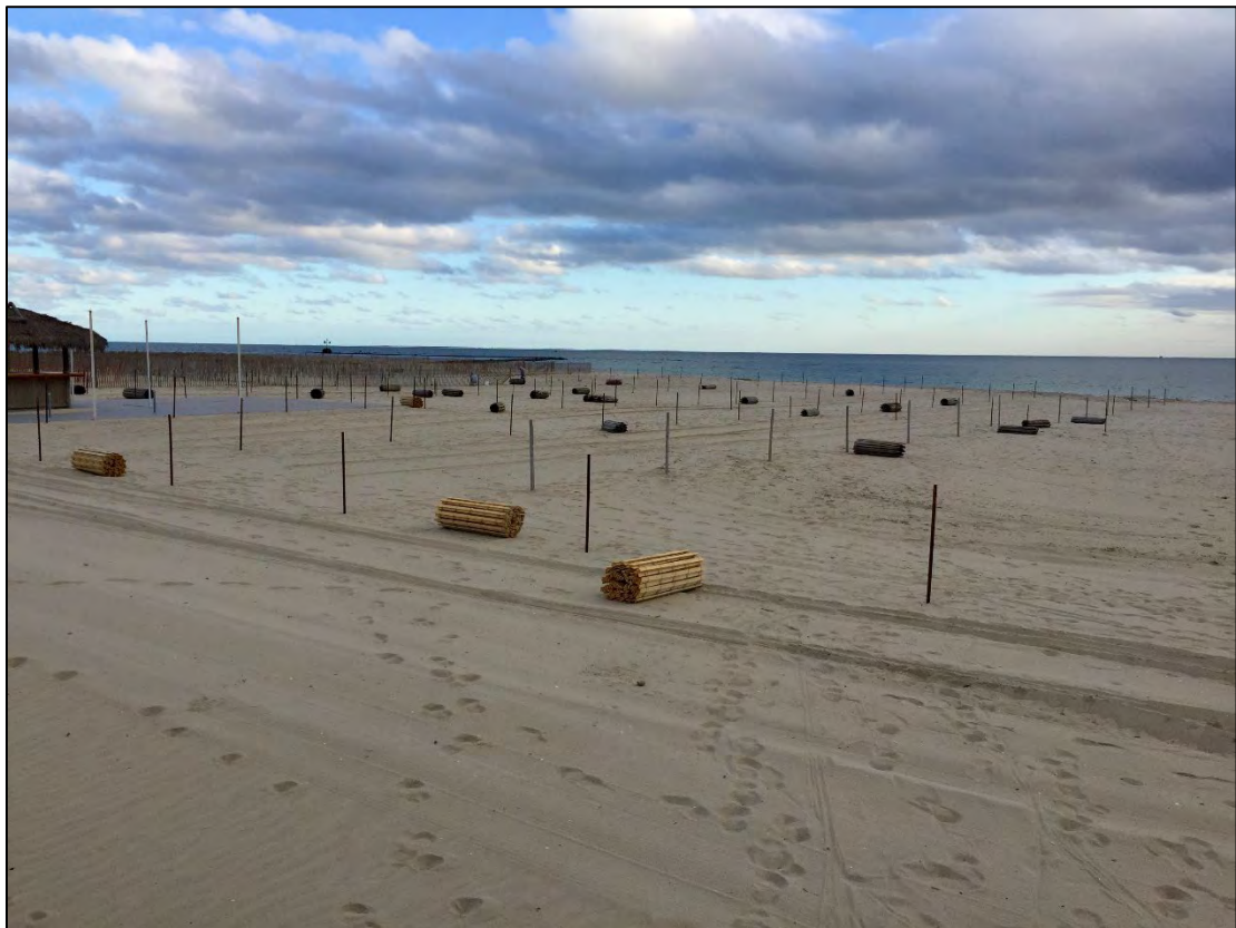
Photo 10: Detail of snow fence installation in November of 2017. Photo courtesy of Wychmere Beach Club (October 12, 2022).
