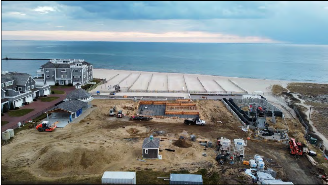
Photo 9: Aerial view facing south of deployed winter snow fencing on the beach and beach club construction in January 2021. Photo courtesy of Wychmere Beach Club (October 12, 2022).
