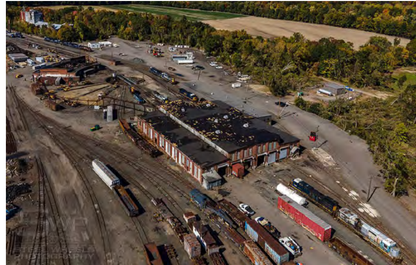
East Deerfield Engine House
