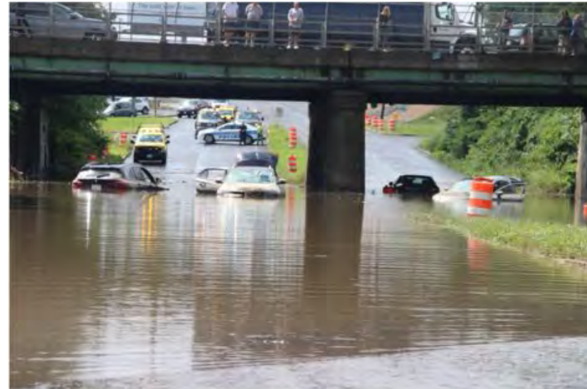
Candidate project under development: flood relief on Route 20/Route 122 interchange, Worcester
