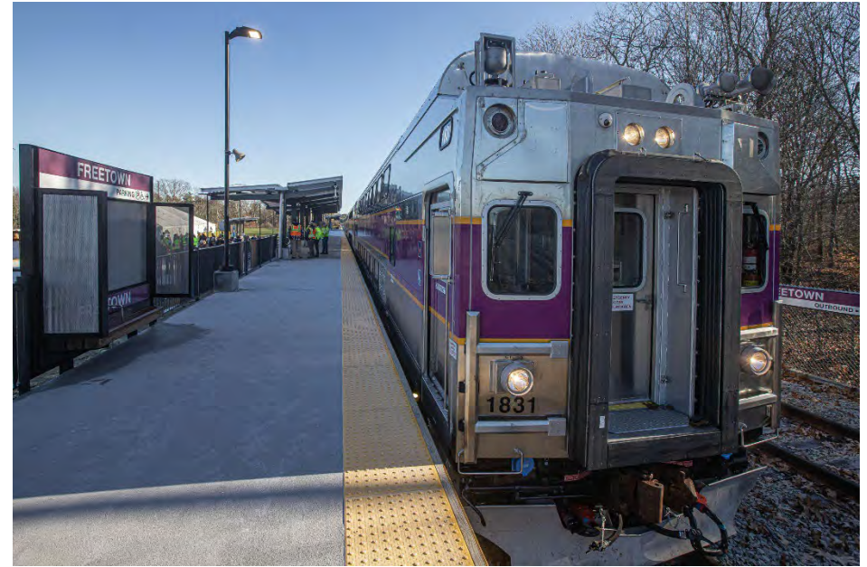
A Commuter Rail coach at Freetown Station during the ribbon-cutting celebrating the substantial completion of the Fall River Secondary Line contract (December 2022)
