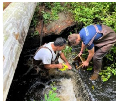
Figure 52. A notch is cut to improve fish passage at the Acushnet River dam in Acushnet.
