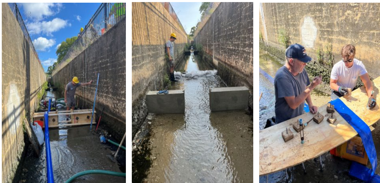
Figure 53. Replacing a weir in the Canal fishway in the Monument River, Bourne.
