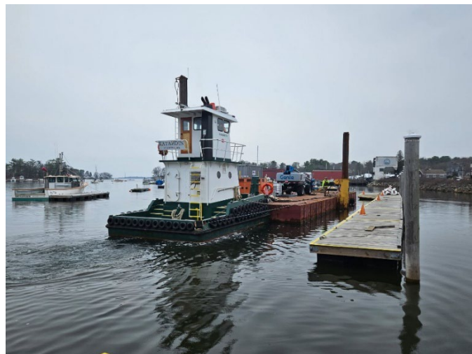
Figure 57. Barge installs Manchester by the Sea transient boater floats and piles funded by DMF's MassBIG .
