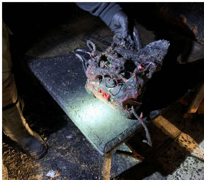
A lithium-ion battery found at the scene of a 2024 fatal fire.
