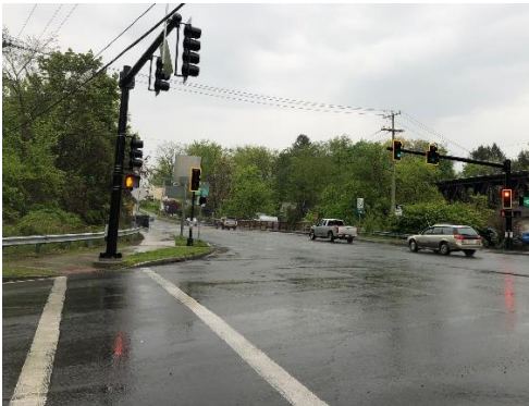
Figure 7 Standard crosswalk (outside of school zone)
