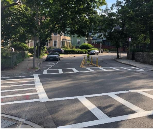
Figure 5 Thermoplastic high visibility crosswalks
