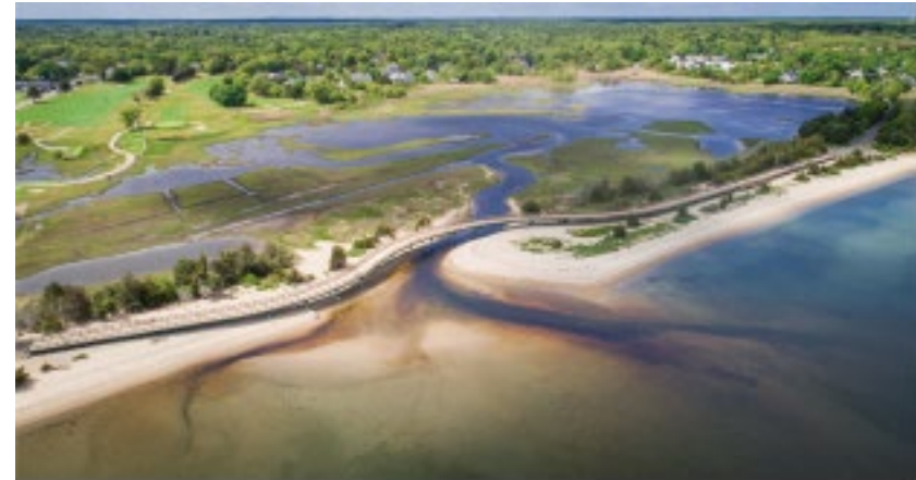
Shining Tides Rail Trail Extension in Mattapoisett
