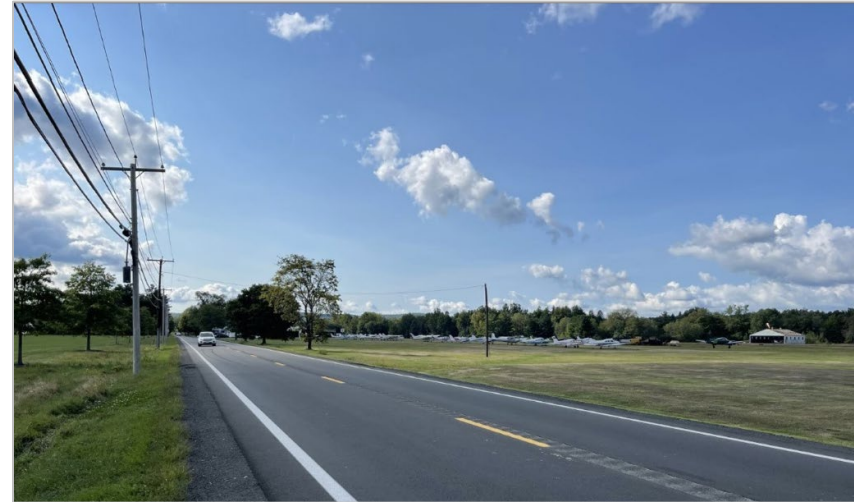
Pavement improvements in Great Barrington
