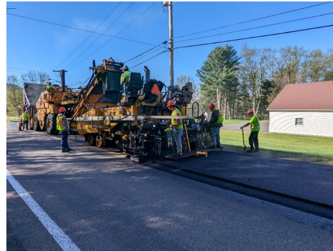
Paving equipment on local roadway
