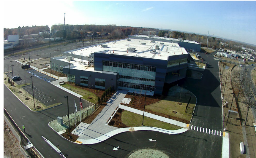
Pioneer Valley Transit Authority Maintenance Facility
