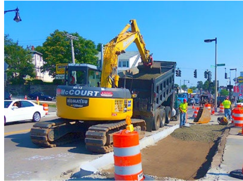
Roadway paving equipment
