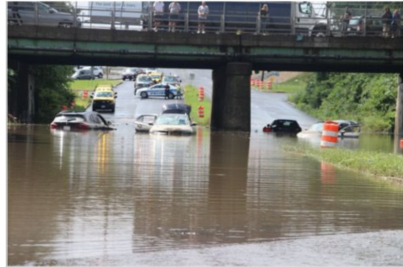
Resilience project location —Route 20/ Route 122 interchange, Worcester
