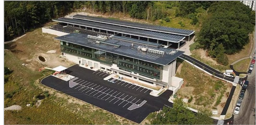
MassDOT Highway District 3 Office
