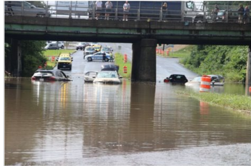
Resilience project location —Route 20/ Route 122 interchange, Worcester
