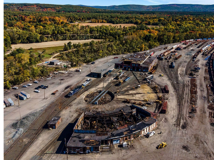
Maintenance yard for track work in Deerfield, MA
