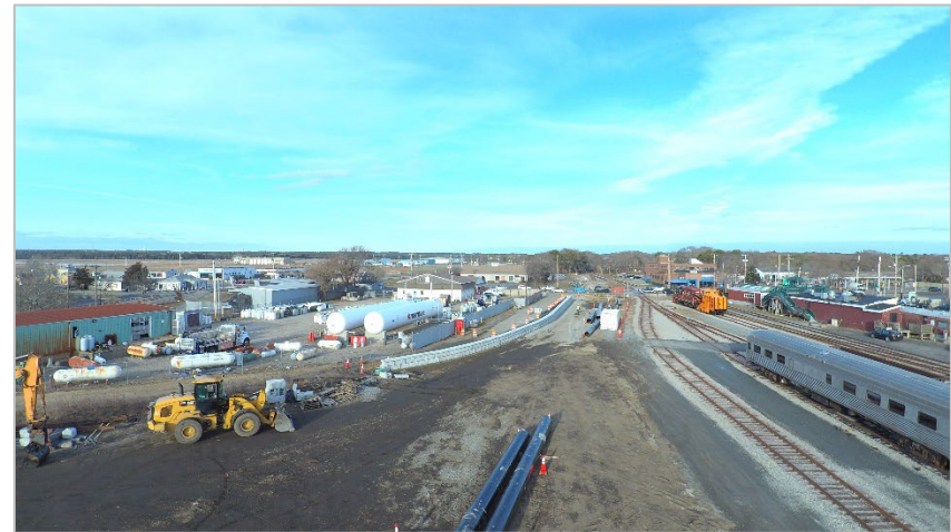
Hyannis Yard on the Cape Main Line
