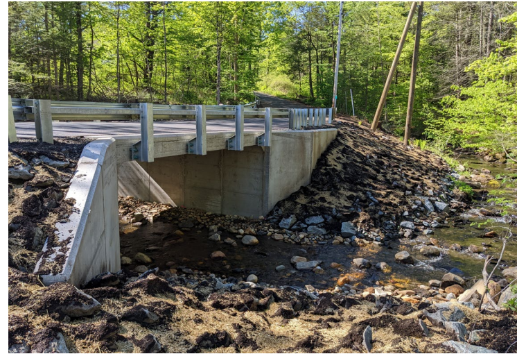
Example of a small bridge
