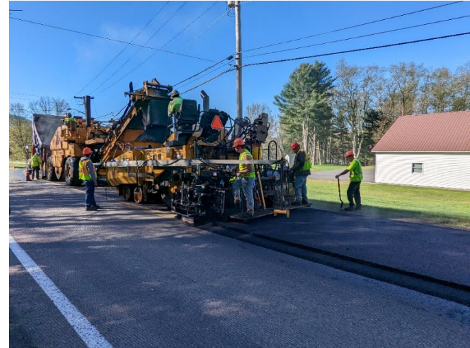
Paving equipment on local roadway
