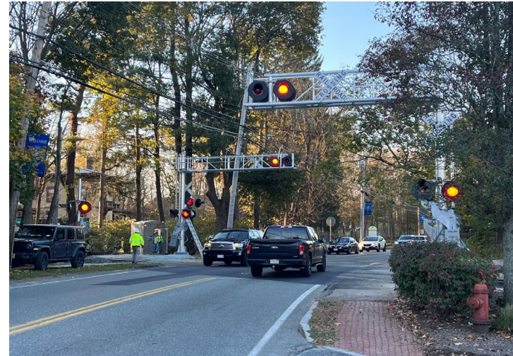
Crossing signal upgrades in Sherborn
