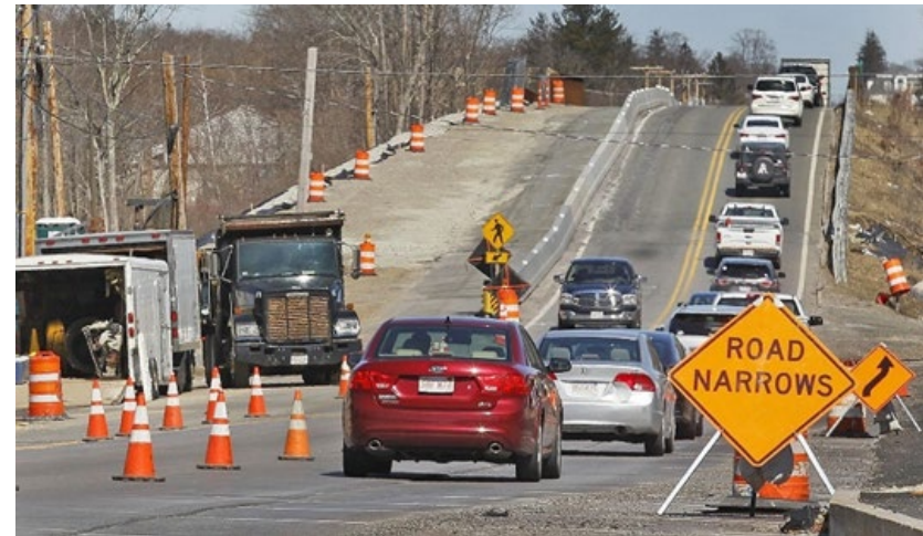
Improvements to Route 18 Weymouth
