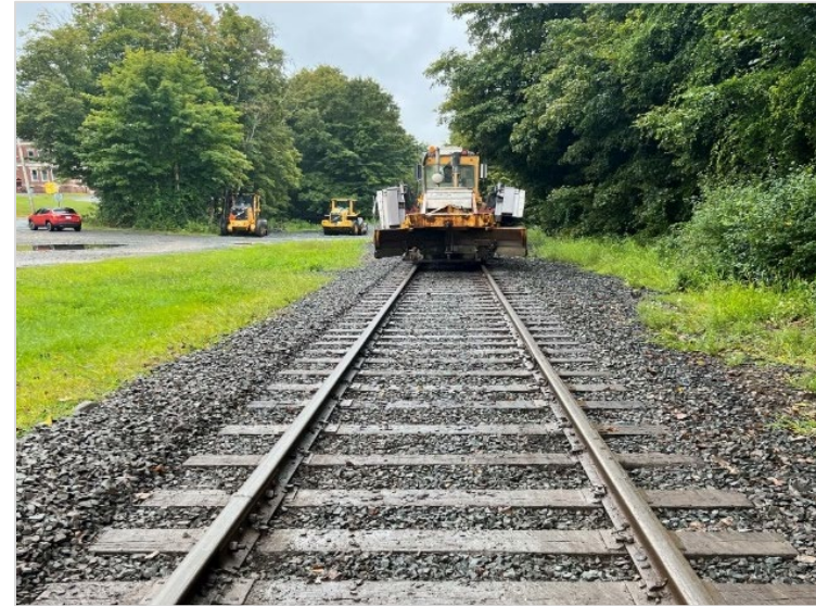
Ballast regulator operation on rail line
