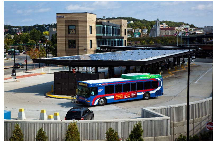
Union Station Bus Transfer Facility in Worcester
