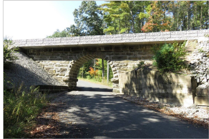
Rail bridge arch deck concrete repair
