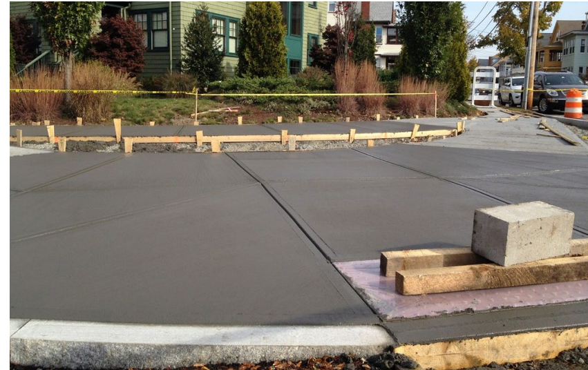
Curb cut improvements
