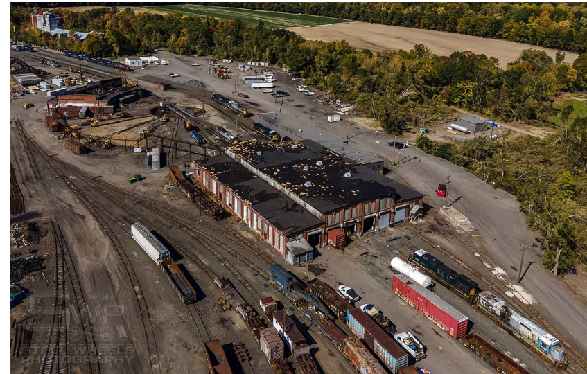
East Deerfield Engine House
