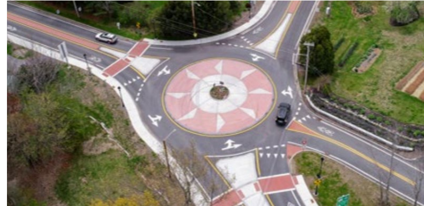
Roundabout on Route 140, Princeton
