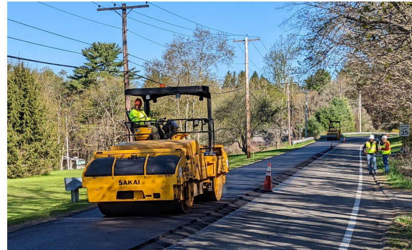
Paving equipment on local roadways
