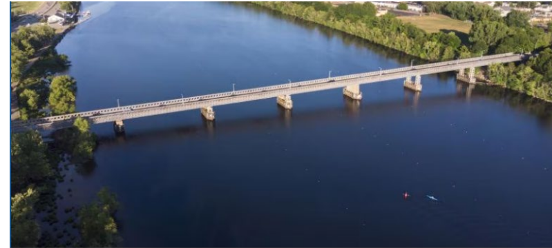
Rourke Bridge in Lowell
