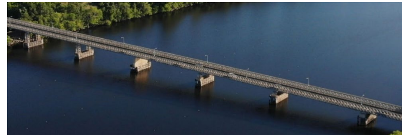
Rourke Bridge in Lowell
