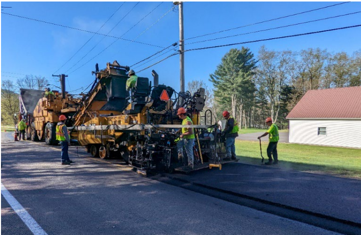
Paving equipment on local roadway
