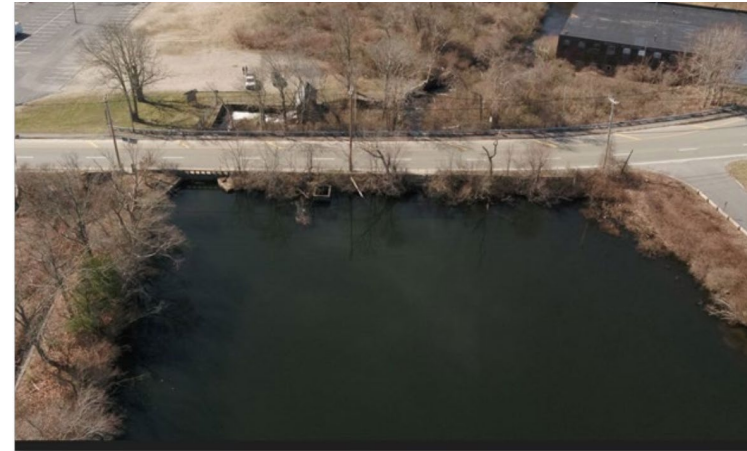
Project: Dam Replacement on Route 28 in Wareham
