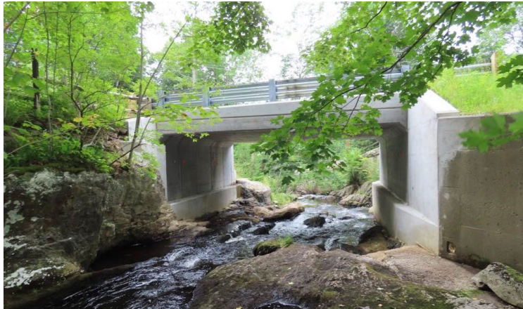
Municipal bridge improvement project
