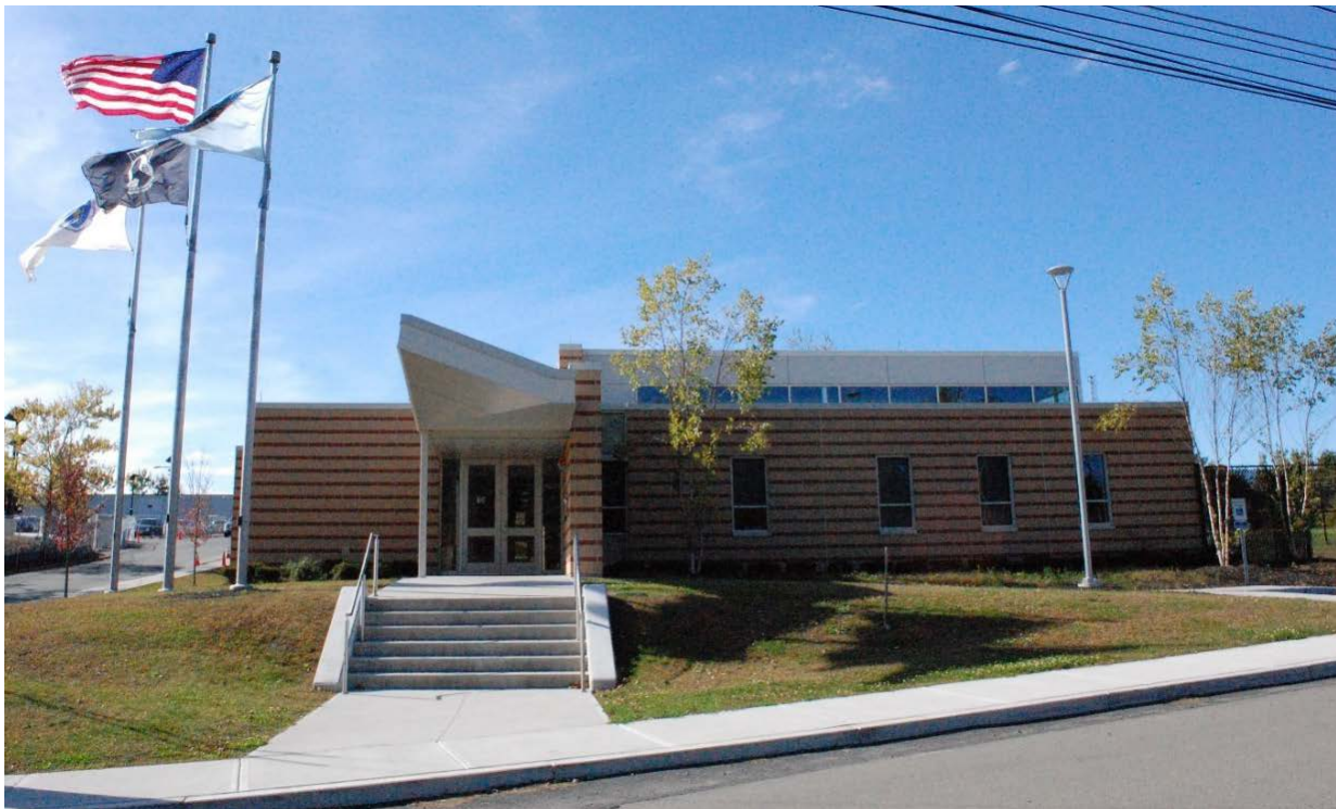
Image 1: North Shore Regional 911 Center
