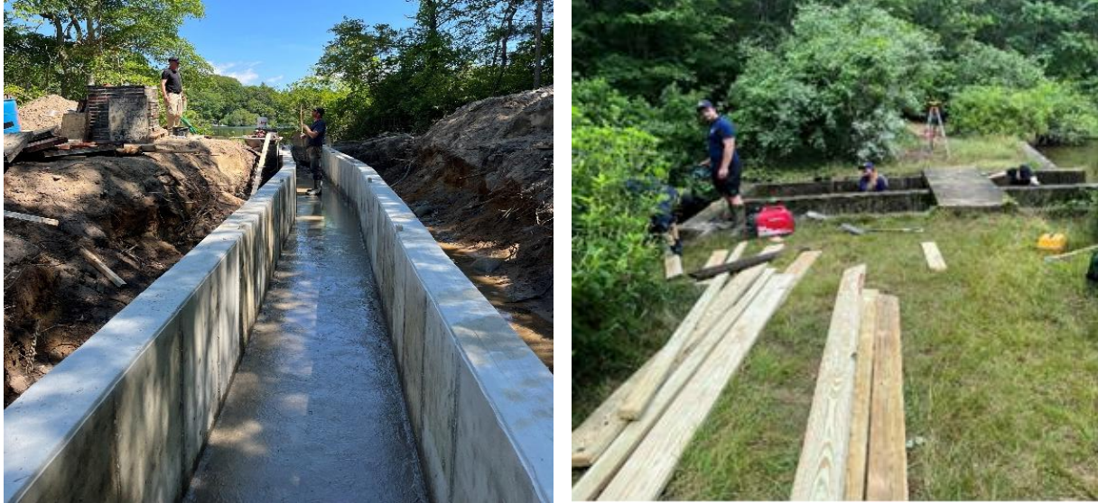
Figure 42. Two DMF Fishway Crew diadromous passage restoration projects in 2025. (Left) Installation of a new daylighted fishway at Bourne Pond, Falmouth; (Right) Repairs to Hinckley Pond fishway on Herring River, Harwich.
