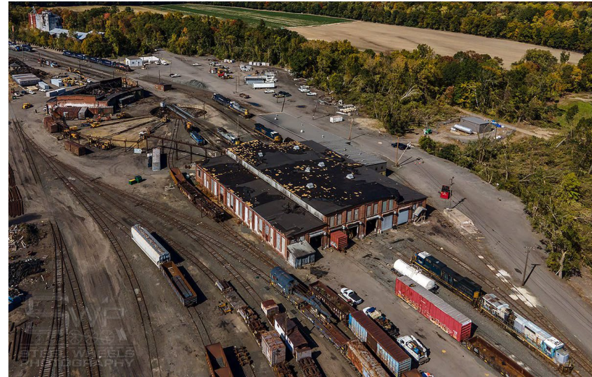
East Deerfield Engine House
