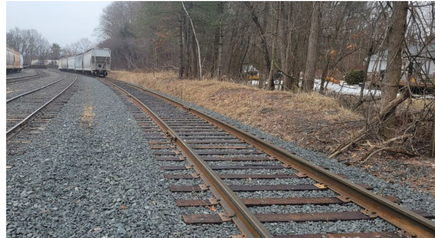
Pioneer Valley Railroad, Easthampton Yard track
