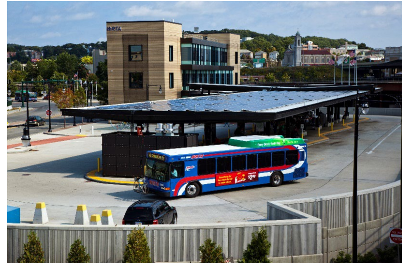
Union Station Bus Transfer Facility in Worcester
