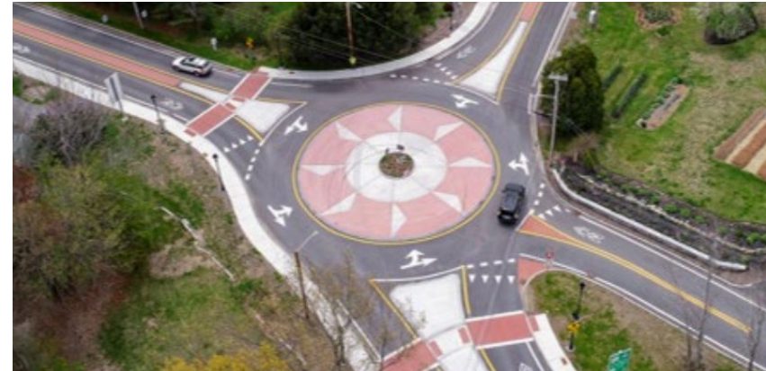
Roundabout on Route 140, Princeton
