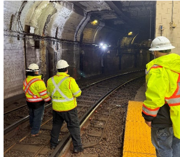
Team performing tunnel inspection using drones
