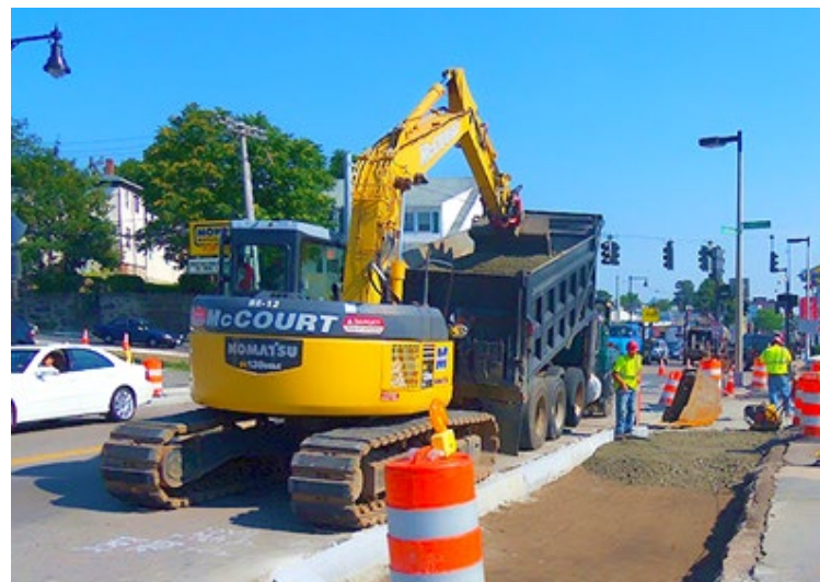
Roadway construction equipment
