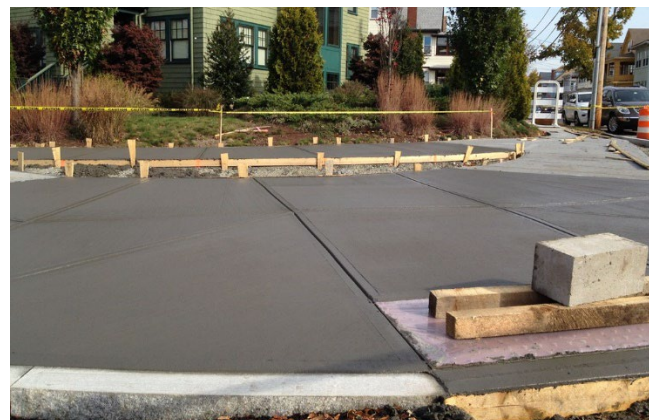
Curb cut improvements
