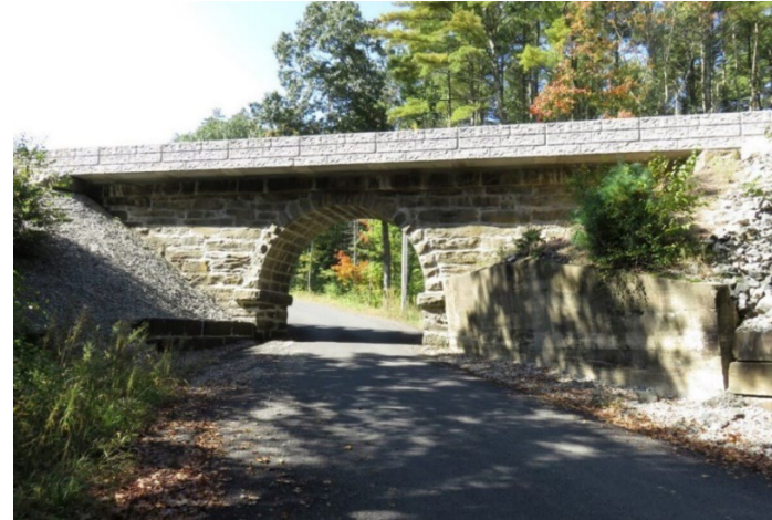
Rail bridge arch deck concrete repair
