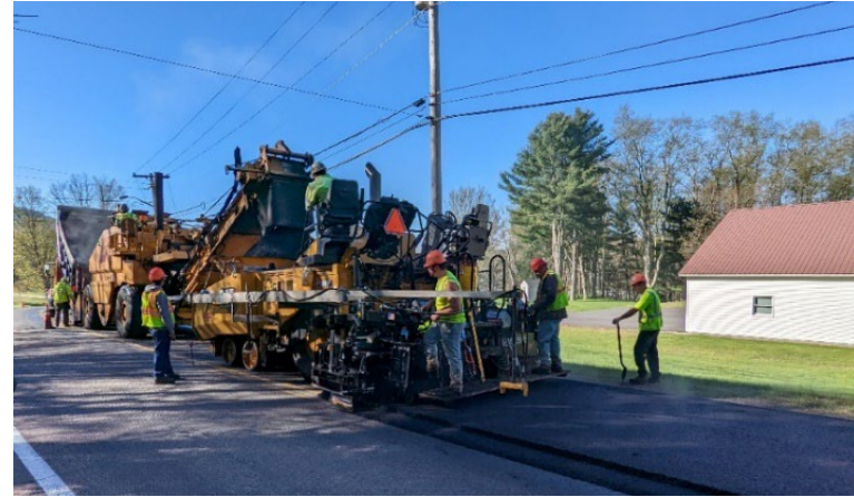
Paving equipment on a local roadway
