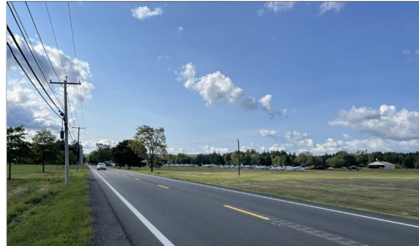
Pavement improvements in Great Barrington
