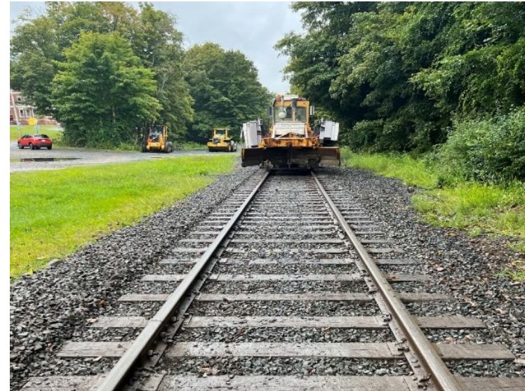
Ballast regulator operation on rail line
