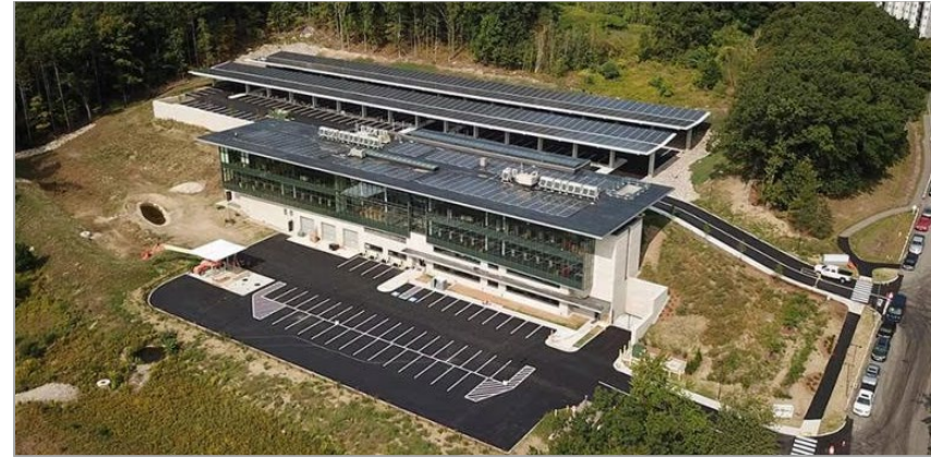
MassDOT Highway District 3 Office
