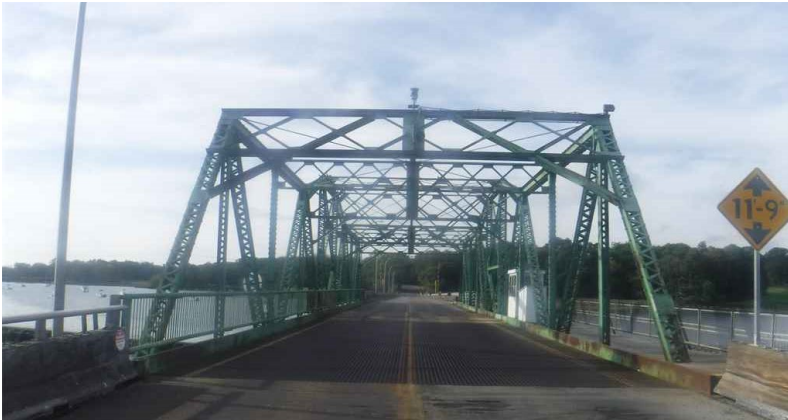
Kernwood Avenue Bridge, connecting Beverly and Salem
