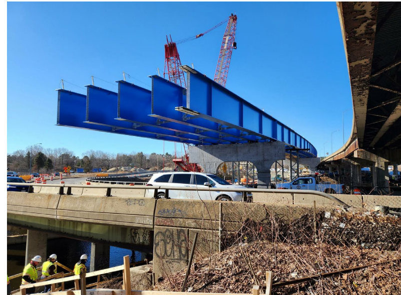
Newton & Weston – I-90 / I-95 Interchange Construction
