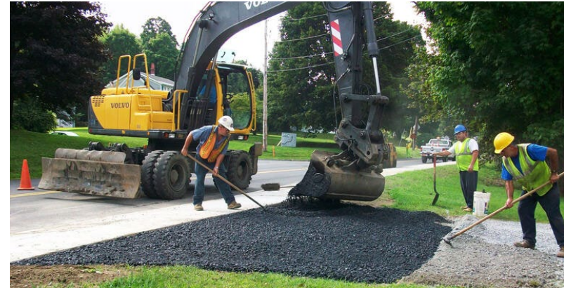
Roadway improvements supported by Chapter 90 funds
