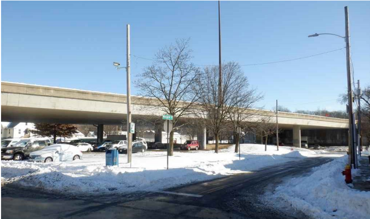
I-391 Bridge over Route 116, Chicopee
