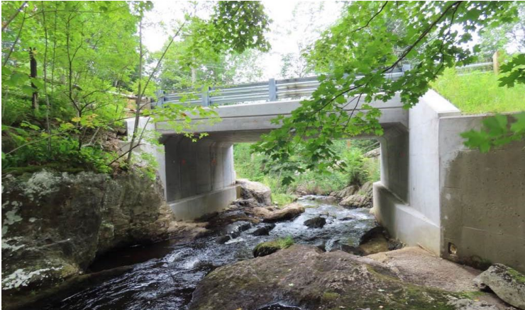
Municipal bridge improvement project
