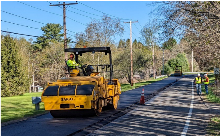
Paving equipment on local roadways
