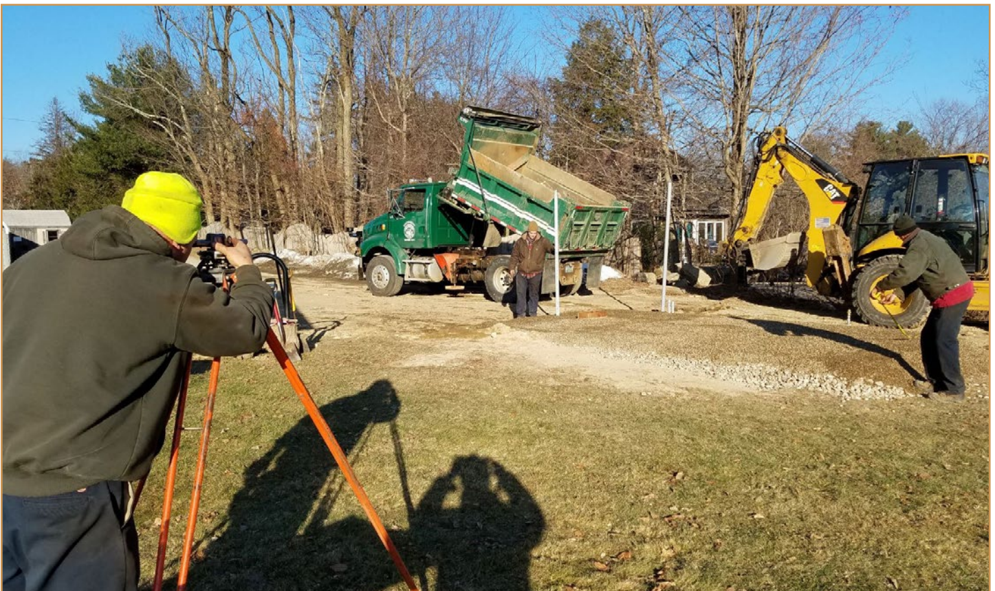
Surveyors leveling the ground to build a central electronics hub for the Town of Shutesbury's municipally-owned fiber-optic network.
