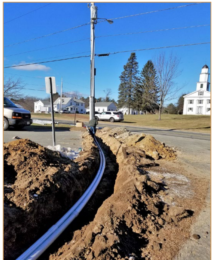
Fiber-optic cable being laid in Shutesbury.
