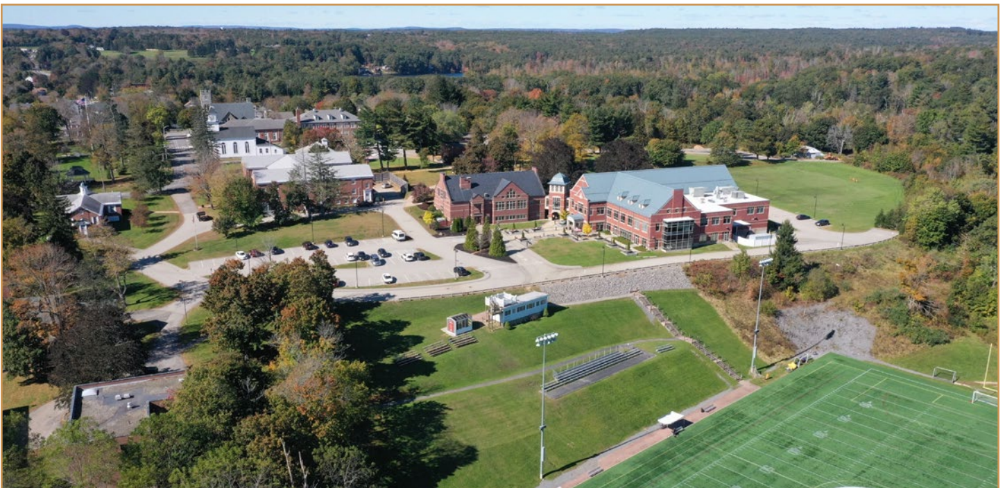
Aerial view of Leicester High School.
