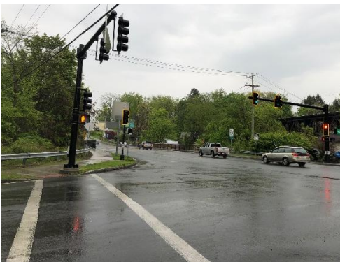
Figure 7 Standard crosswalk (outside of school zone)
