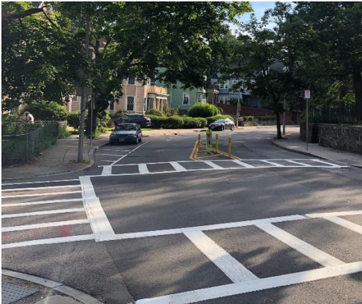
Figure 5 Thermoplastic high visibility crosswalks
