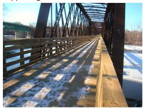
months, DCR's contractor MAS Bridge and Building, has removed the old decking and railings, replaced railroad ties, and in nearing completion on re-decking the bridge. They expect to wrap up this phase in March, and then complete repairs to the steel structure and stone piers by the end of April. DCR hopes to then reconstruct the Damon Road Parking lot by early summer.
