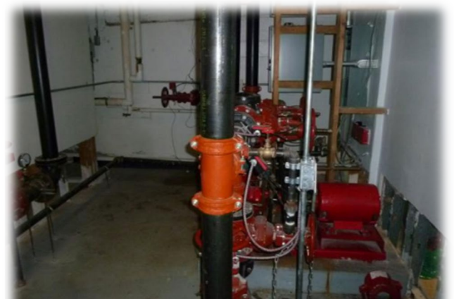
Wet Sprinkler System
