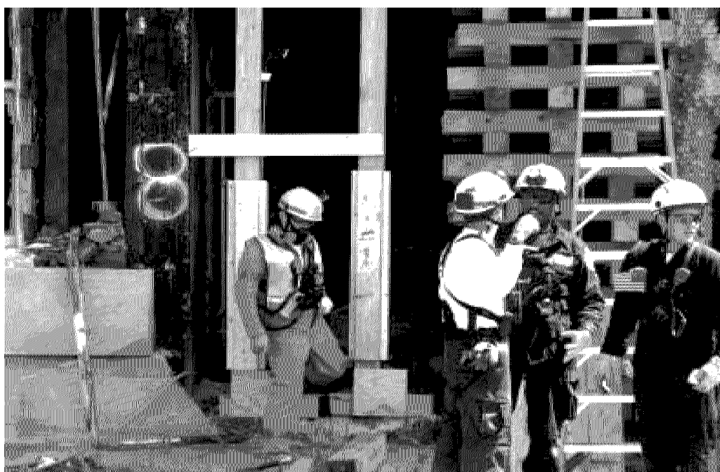
US&R shoring and marking system.
