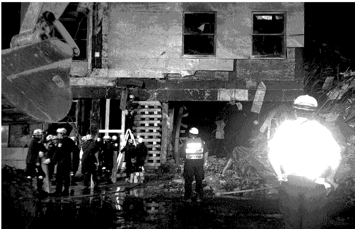
Figure 16. Start of shoring operations. Photo taken as the first crib shore is being completed at approximately 1:00 a.m. the morning of September 12 th , 2001.
