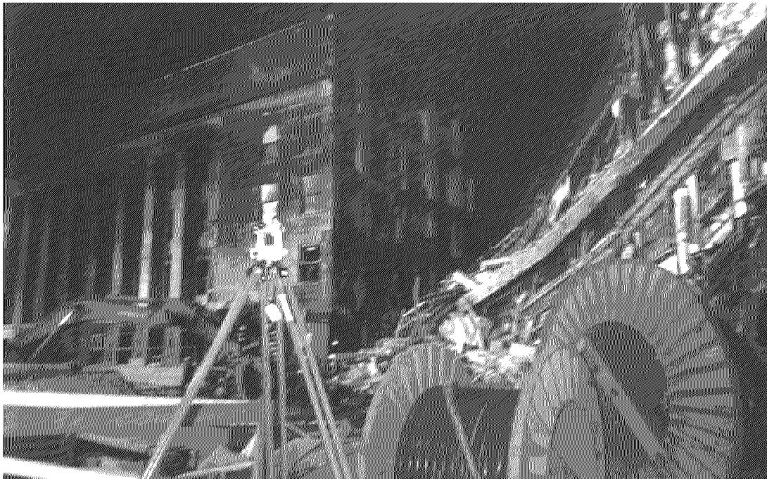
Figure 15. Transit monitoring station. Transits were set up to monitor several points on the building during the shoring operations.
