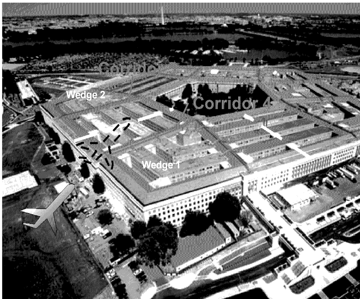
Figure 4. Approximate location and angle of impact and its relationship to Wedge 1 and Wedge 2 (Tills, 2001)
