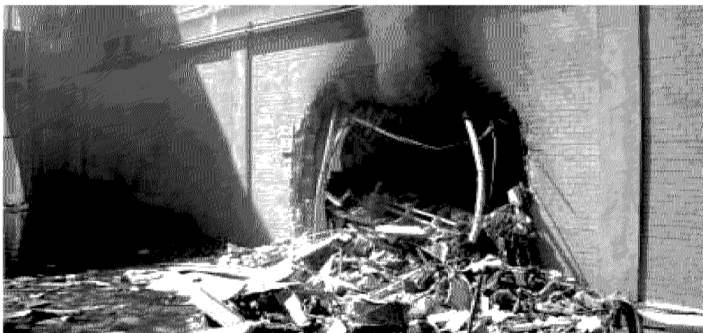
Penetration through the inner wall of the Pentagon's C Ring.
