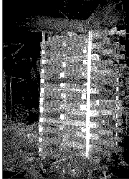
Figure 19. 9 point crib shore. Used where columns were severely damaged or missing completely.
