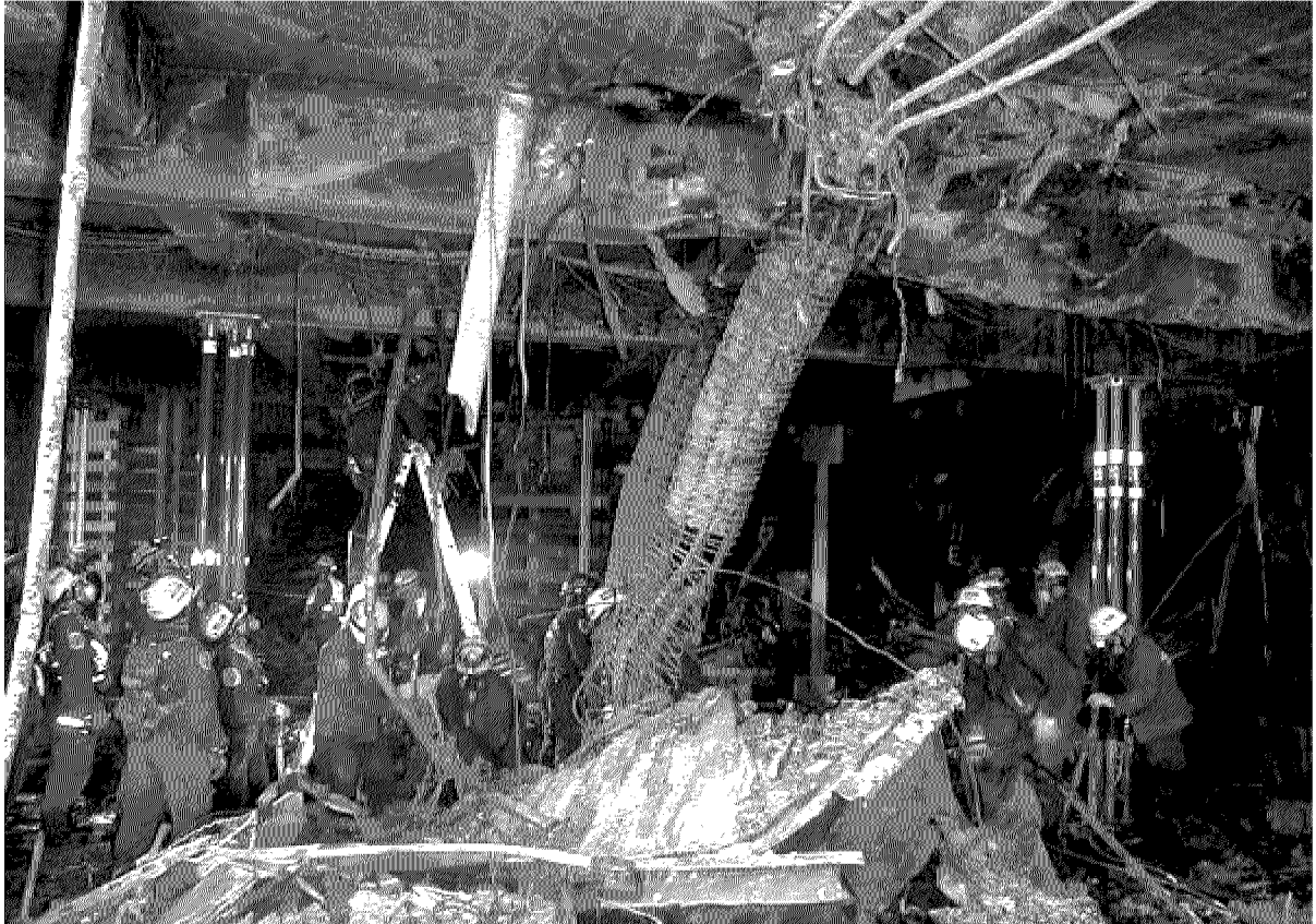
Figure 12. Internal damage to concrete columns and beams.
