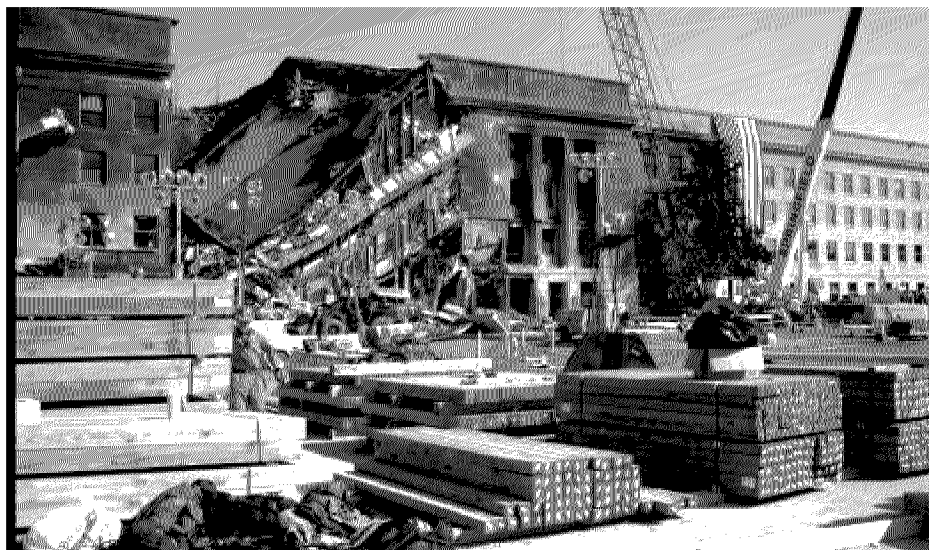
Figure 17. Lumber storage. Lumber for shoring was delivered to the site by Home Depot and stored on the concrete helicopter pad.
