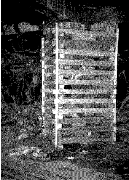
Figure 18. 4 point crib shore. Used to support damaged columns still carrying loads.
