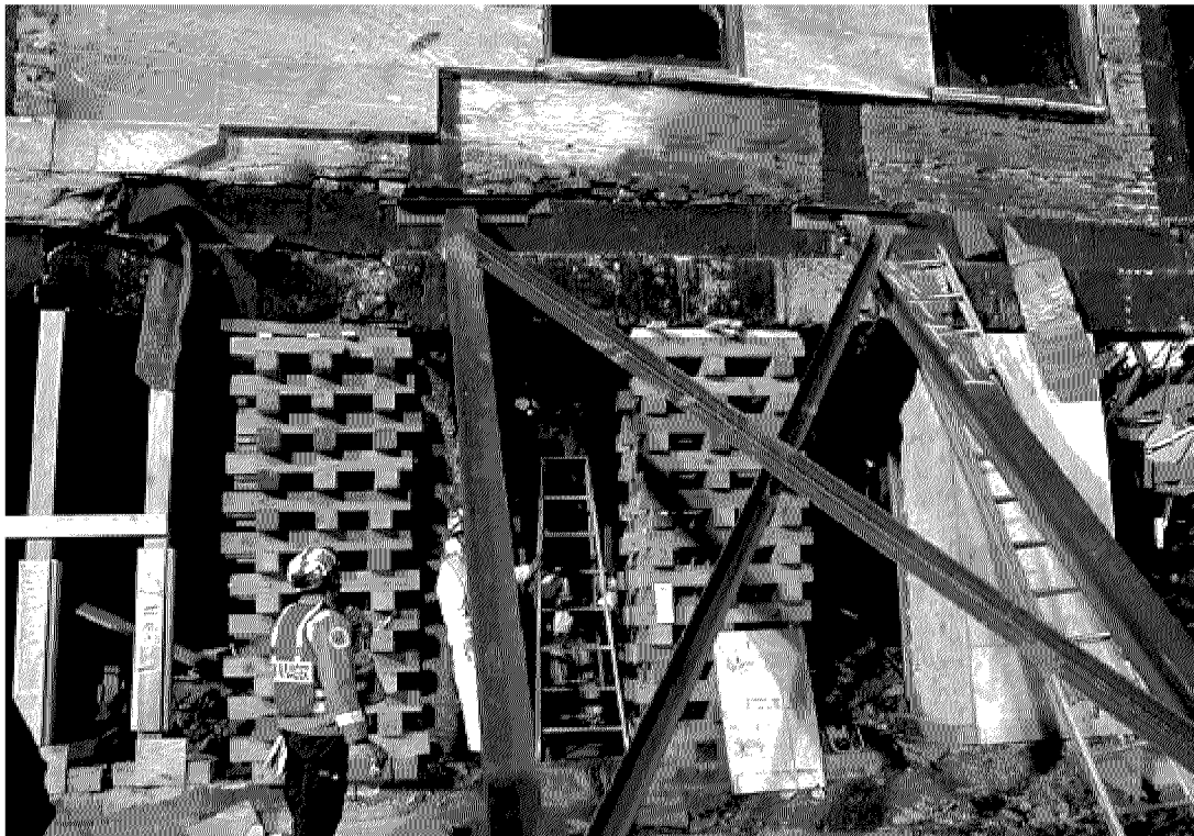
Figure 23. Raker Shore for lateral support. Notice the 3 crib shores and 2 vertical post shores for vertical support. The shims at the top of the crib shore were over-tightened causing the concrete beam to shift slightly. VA-TF1 Structural Specialist section leader, Dean Tills, is standing to the left of the raker shore.
