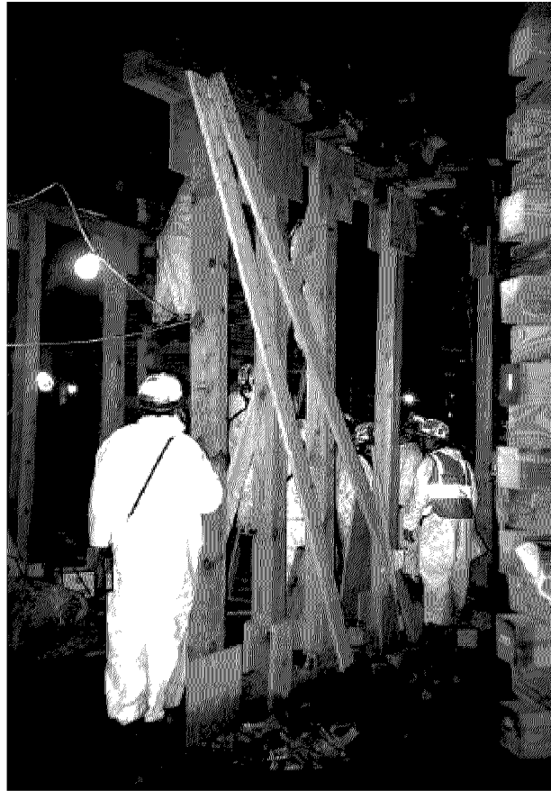
Figure 22. Vertical shores.
