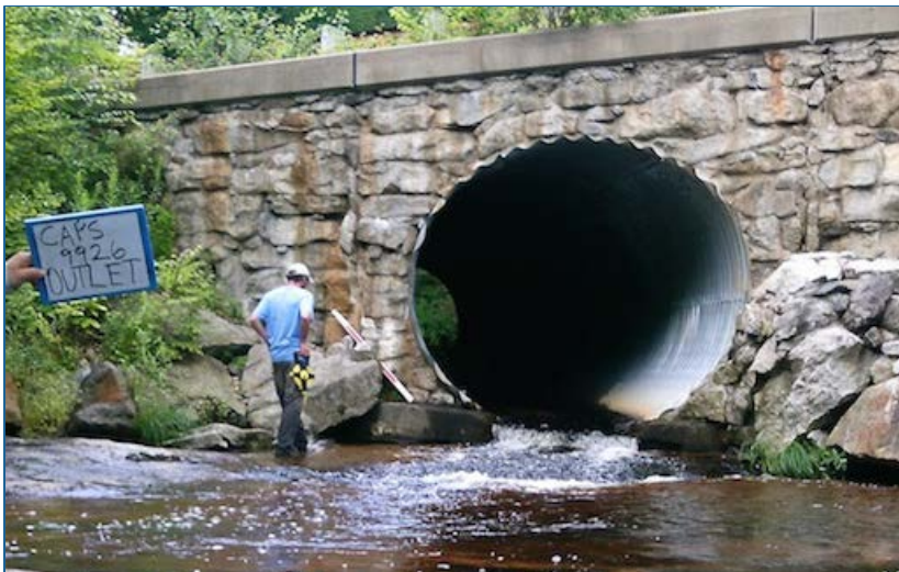
Figure H-5: Culvert 9926 inlet (top) and outlet (bottom) with a diameter of 10 ft on both sides.
