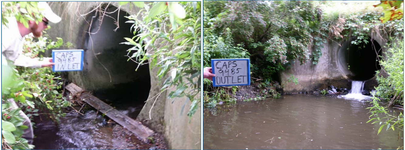
Figure H-3: Culvert 9485 inlet and outlet. The inlet (left) has a diameter of 4.5 ft. The outlet (right) has a diameter of 5 ft.
