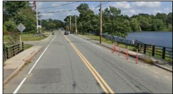
Central Street Bridge
