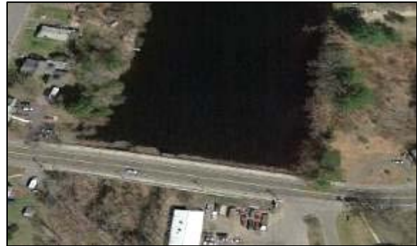
Island Grove Pond Dam, located at the southern end of the pond at Centre Ave. (Rt. 123)
