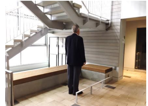
Lack of protection underneath stairs
