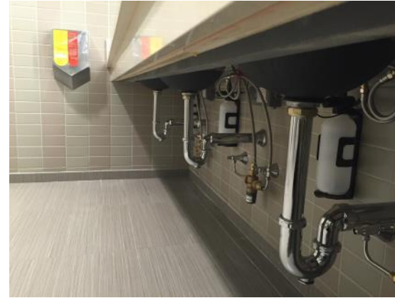
Lack of protection underneath sink
