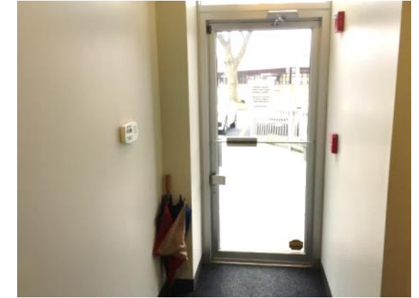
Lack of maneuvering clearance at door
