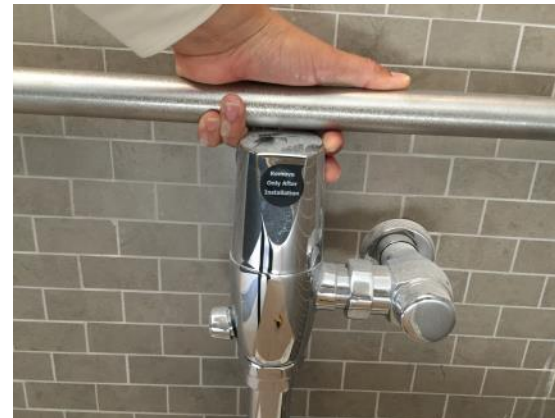
Rear grab bar obstructed by flush valve
