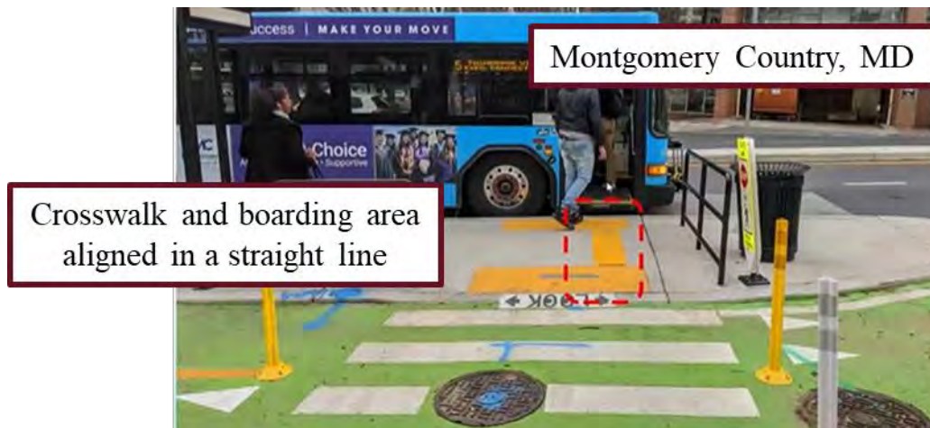
Figure 4.15: Crosswalk, tactile pavement, and boarding area aligned in a straight line
