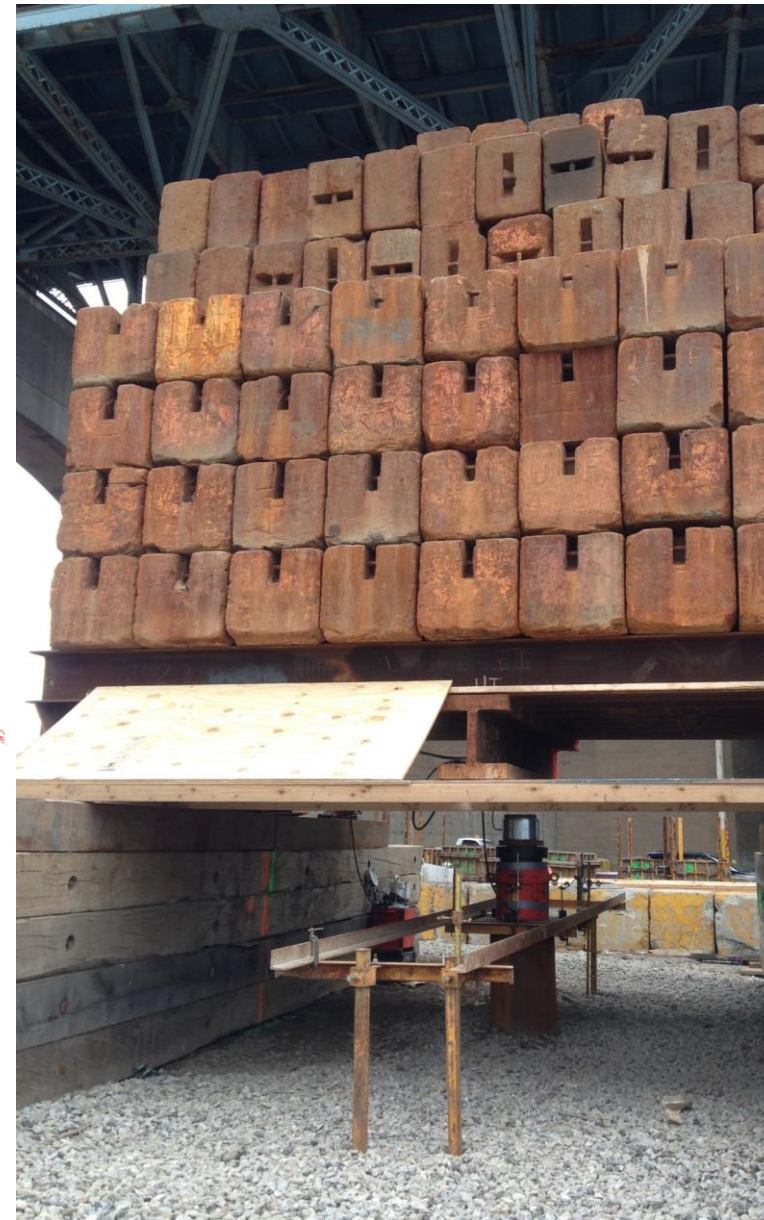
Example Pile Load Test
