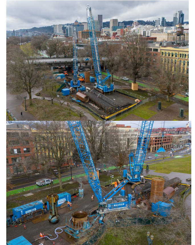
Example Drilled Shaft Load Test
