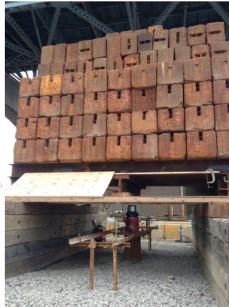
Example Pile Load Test
