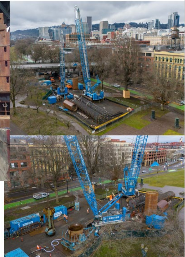
Example Drilled Shaft Load Test
