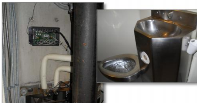
Sheriff's Departments. in Middlesex, Plymouth and Essex Automated water management system for lavatories
