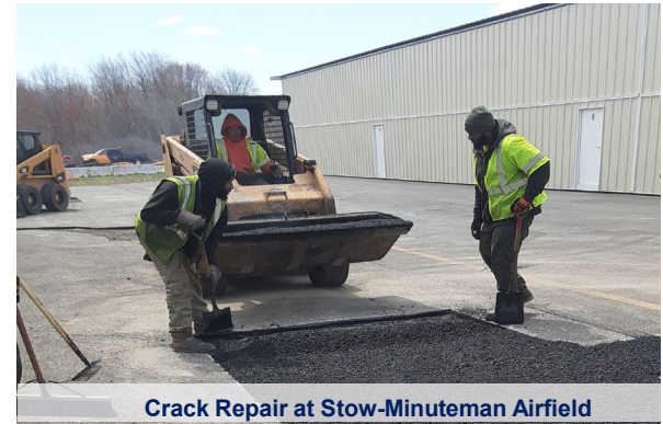
Crack Repair at Stow-Minuteman Airfield
