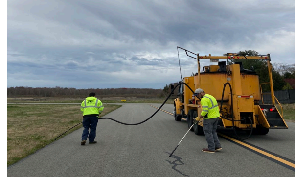
Crack Sealing at Marshfield Municipal Airport
