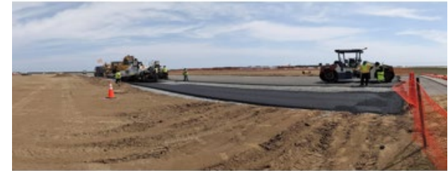
Paving Crew begins placement of Airfield Bituminous Pavement
