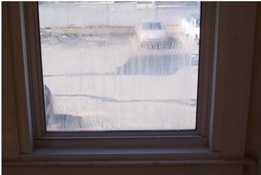
Unit 8A Window Condensation
