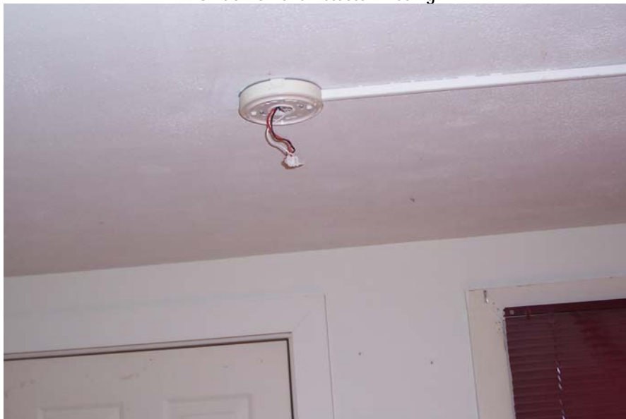
Unit 8A Smoke Detector Missing
