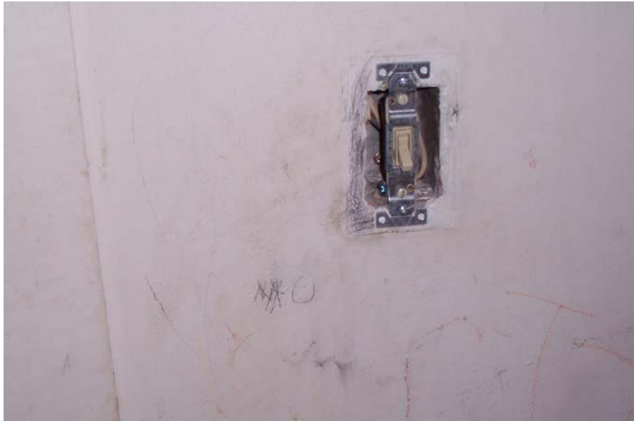
Unit 1B Switch Plate Missing
