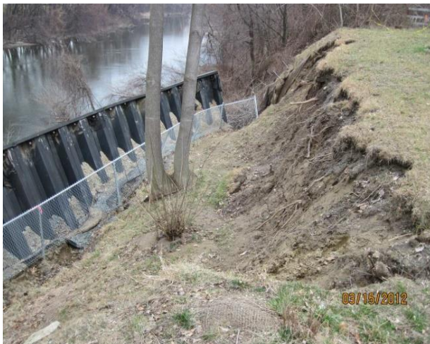
Hurricane Irene caused sheet piling in a 250' section of levy along the Westfield River to erode and fold.
