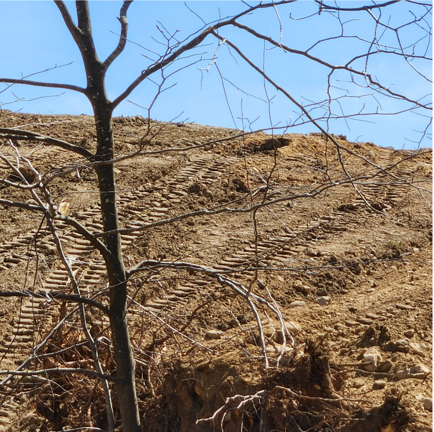
Clearing the trees
