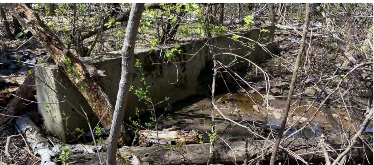
Outfall for Stormwater Collection from Roadways
