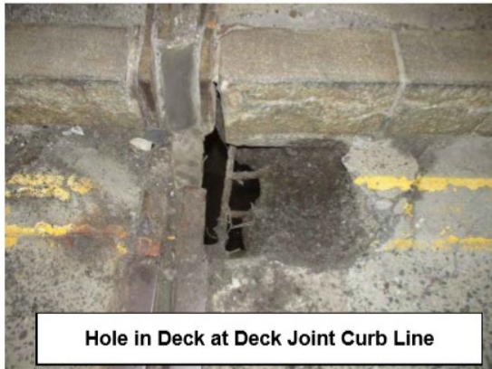
Corrosion of SIP Forms/Exposed Deck Rebar
