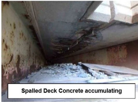
Hole in Deck at Deck Joint Curb Line
