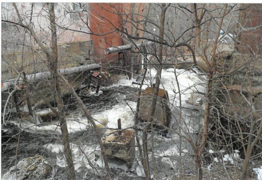
Deteriorating, asbestos-covered pipe poses a contamination risk, should future severe storms and Powwow River flooding cause supporting structures to collapse.
