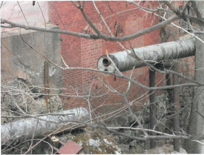
Deteriorating, asbestos-covered pipe poses a contamination risk, should future severe storms and Powwow River flooding cause supporting structures to collapse.
