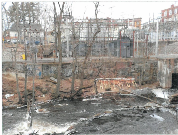
National GRID power station is located on eroding banks of the Powwow River, putting the power station at risk for flood damages.
