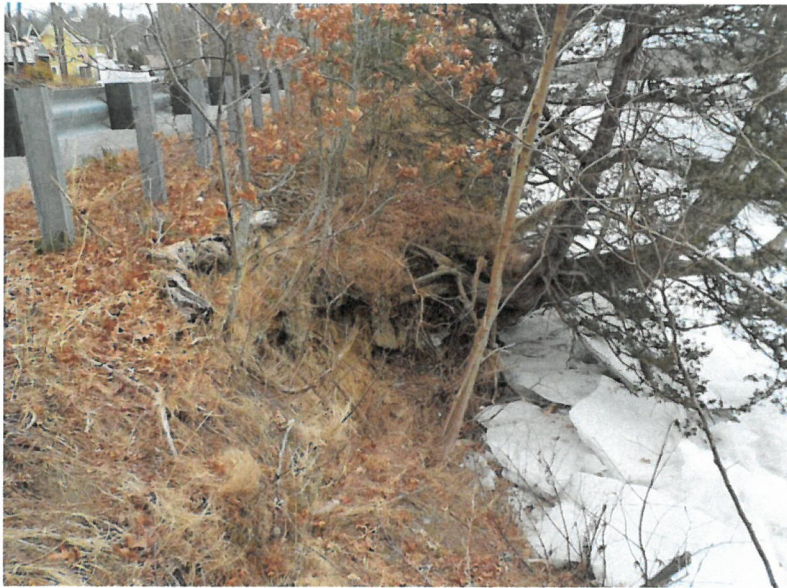
Severe storms, sea level rise, coastal storm surge, winter river ice action, and boat wakes are all contributing to the worsening of erosion of the banks of the Merrimack River at Pleasant Valley Road.
