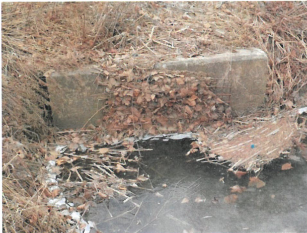
Culvert replacement study could evaluate feasibility of replacing currently clogged and undersized culvert with one that meets Massachusetts stream crossing standards.
