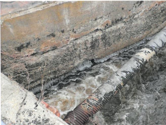
Note river water beneath cement wall.
