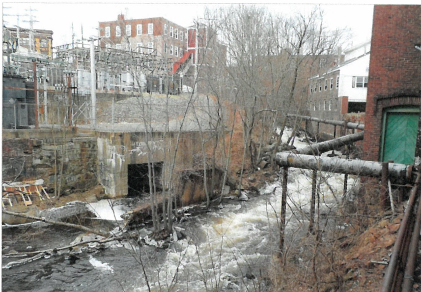
National GRID power station is located on eroding banks of the Powwow River, putting the power station at risk for flood damages. Note asbestos-covered pipe (not part of National GRID site) on deteriorating supports over the river.
