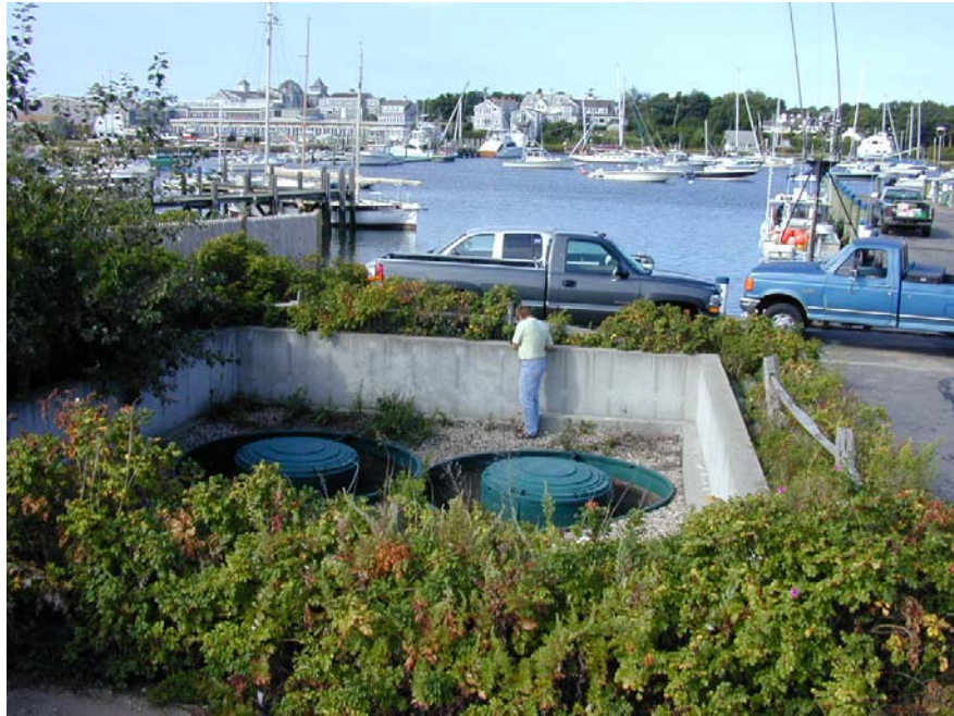
Figure 8. StormTreat™ Installation Site adjacent to the Wychmere Harbor Town Pier parking lot in Harwich.
