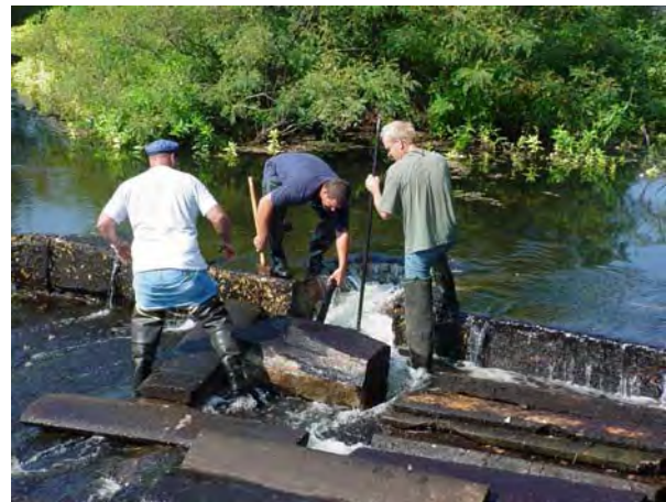
Figure IVC1.3 Notching of Bleachery Dam.
