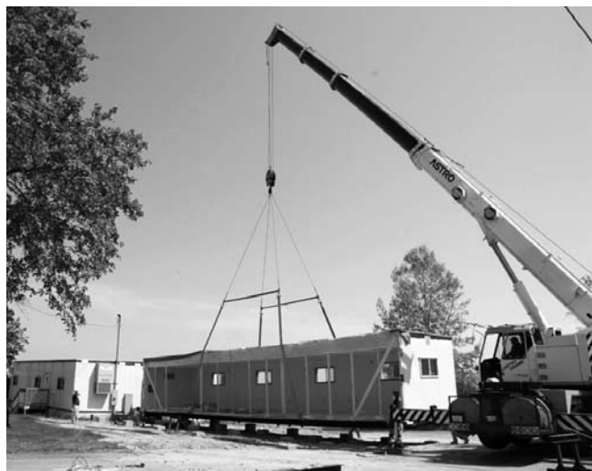
A crane installing Building C at Westborough Field Headquarters.
