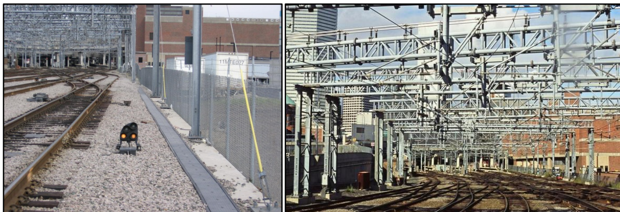
Dwarf Signal at Tower 1 Interlocking
