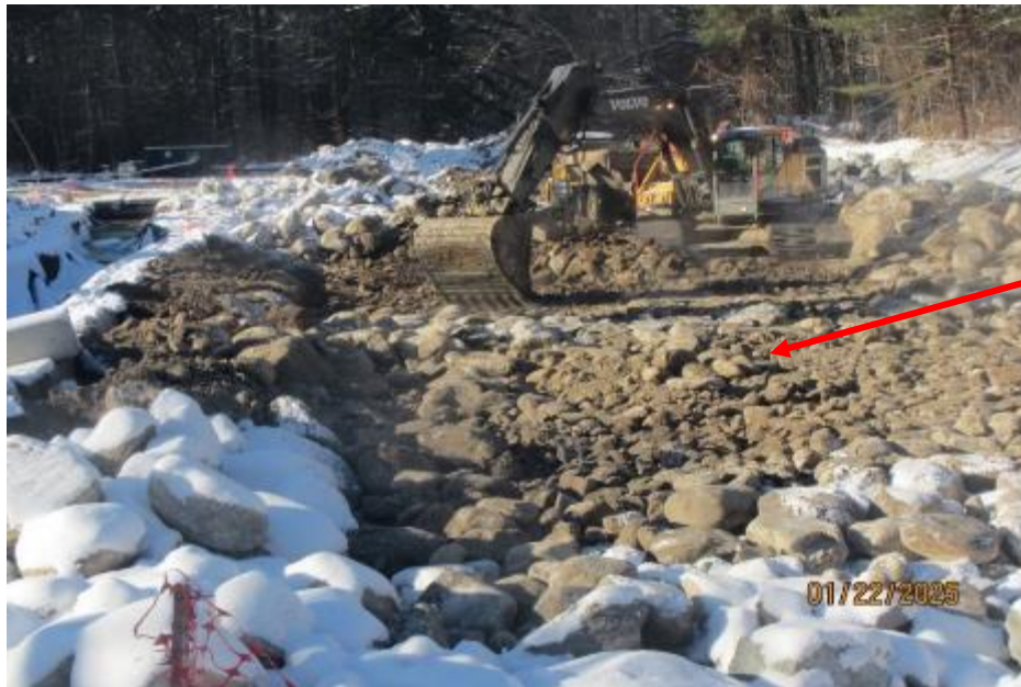
Placement of rock for riverbed riffle
