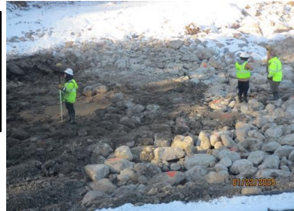
Checking riverbed grades
