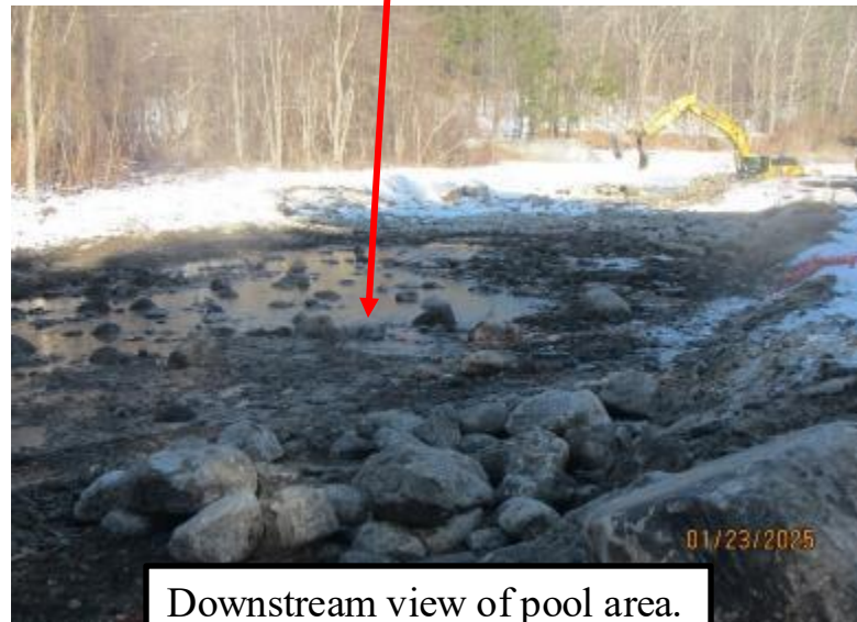
Placement of rock for riverbed riffle
