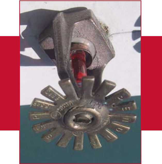
Sprinkler Head. Photo by Jessamyn West.
