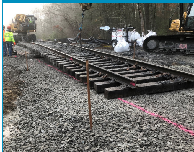
Resetting track panel over culvert in Lakeville
