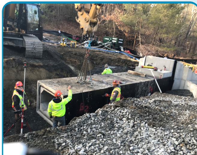
Installing box culverts in Lakeville
