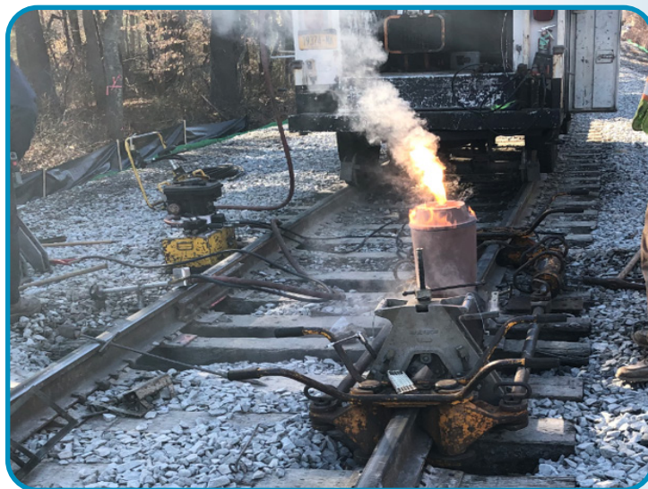
Rail welding at a culvert in Taunton
