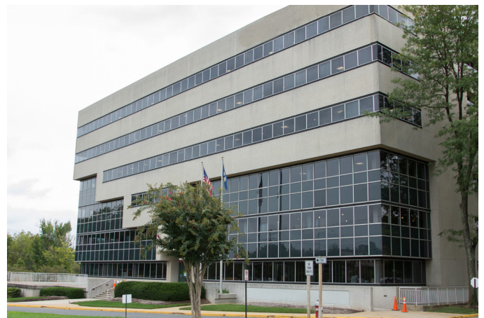
Figure 5: Front and west side of building
